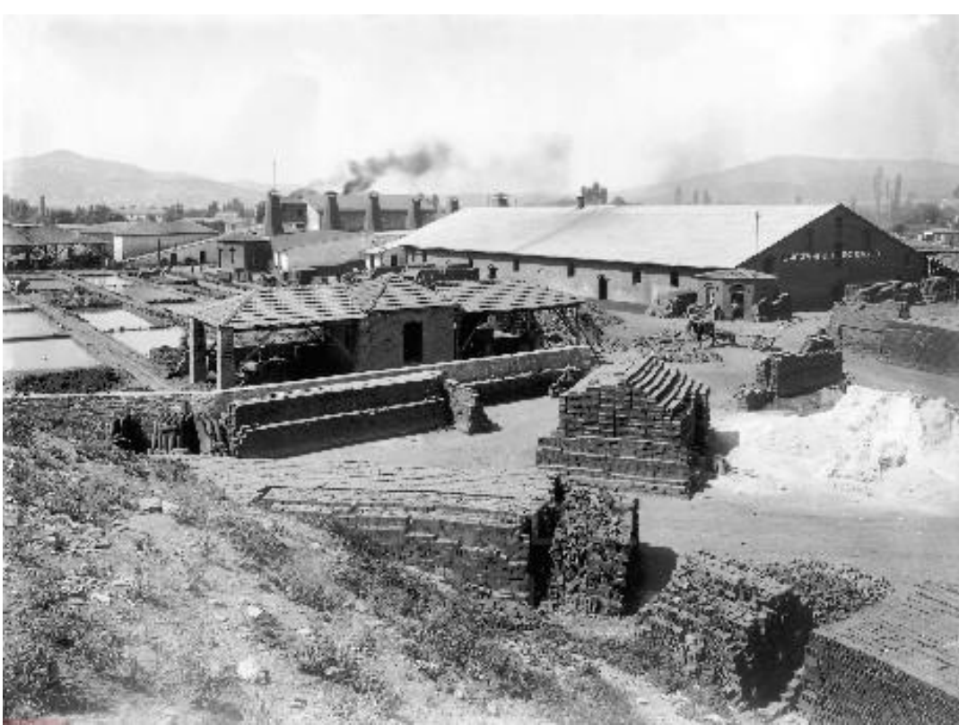
Fig. 48. The Tsalapatas Rooftile and Brickworks Factory – before.
