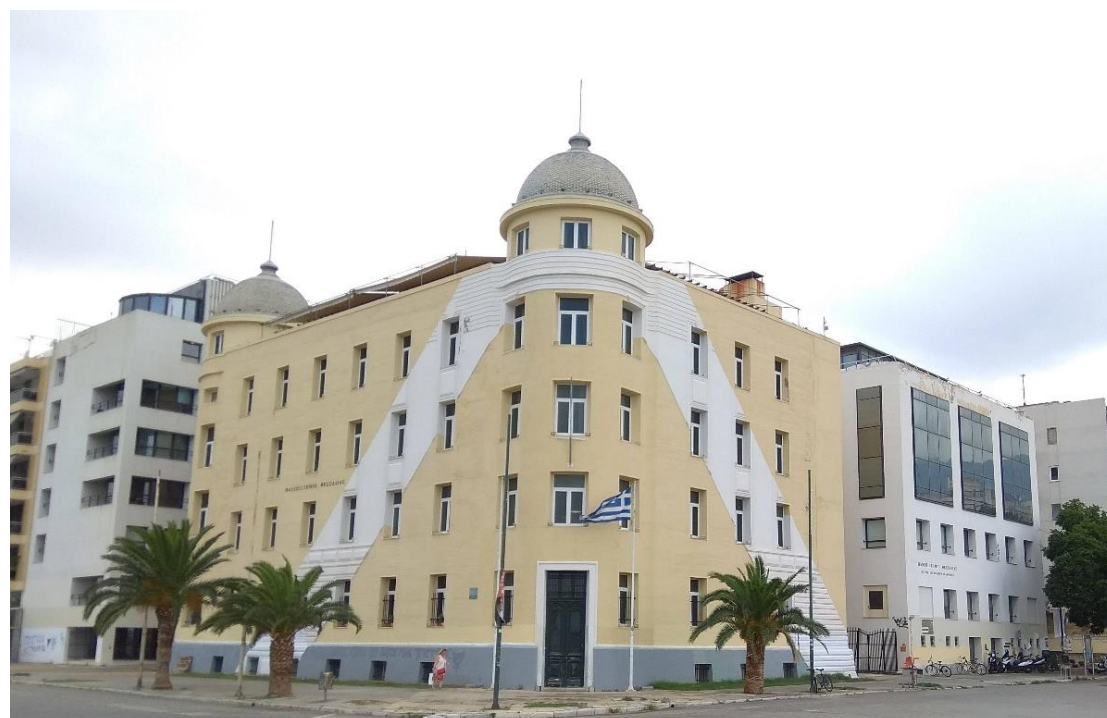
Fig. 45. (down) Papastratos Tobacco Warehouse today houses the Central Administration and the Department of Pedagogy. Photographs below show the remaining decorative features after conversion.
