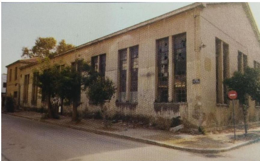
Fig 39. The former Electric Company used nowadays as a Theatre and Municipal Dance School - before and after.
