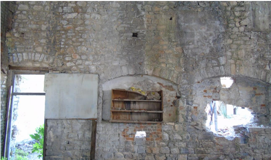
Fig. 13. Foundry Workshop, view from the interior.
