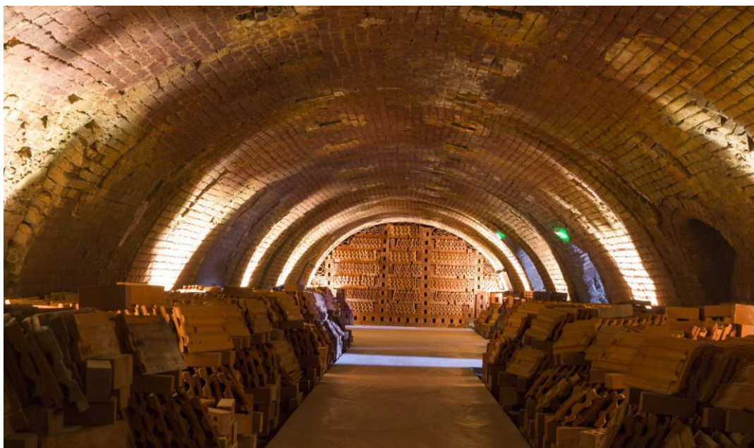
Fig. 50. The imposing Hoffmann kiln remains a factory installation and is among the best-preserved features.
