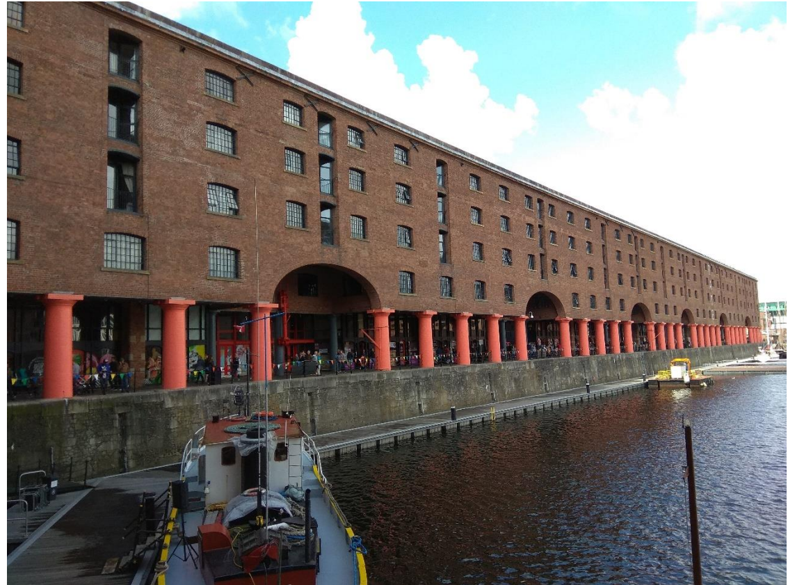
Fig. 54. Conversion of part of one warehouse stack into the Tate Liverpool by James Stirling, Michael Wilford, and Associates.
