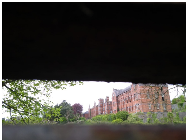
Figure 2: a photograph of the Sundays Well Magdalene institution, taken through a security gate.
