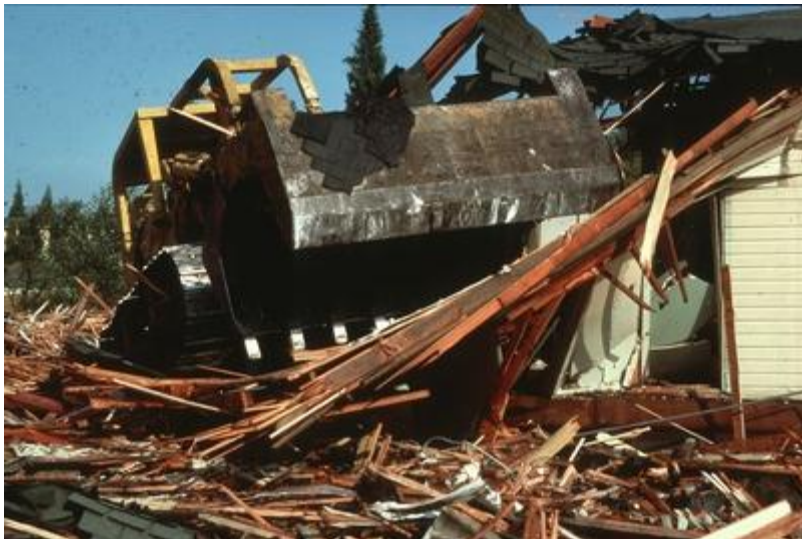
18. Building demolition at Discovery Park. 1980. 460
