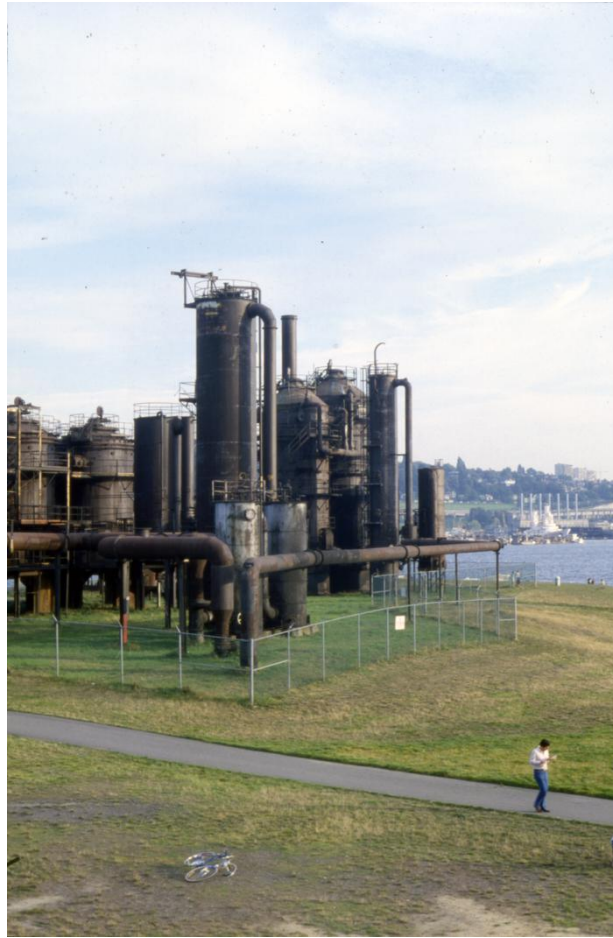
4. Cooling towers retained at Gas Works Park, 1976. 114
