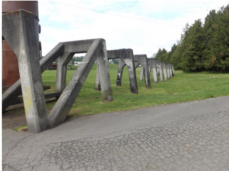
2. Remains of track trestles. April 2016. 88
