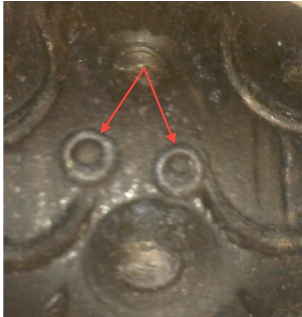
Fig. 4 Two circles made by a tubular drill
