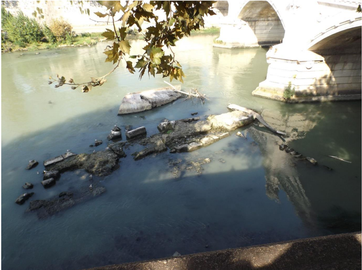
Figure 11 and 12: The visible remains of the Pons Neronianus taken from the east bank of the Tiber. In the lower image the piers of the modern Ponte Vittorio Emanuele II can be seen in the background and the triangle shape of the pier with the triangular end facing toward the river current. Author images.
