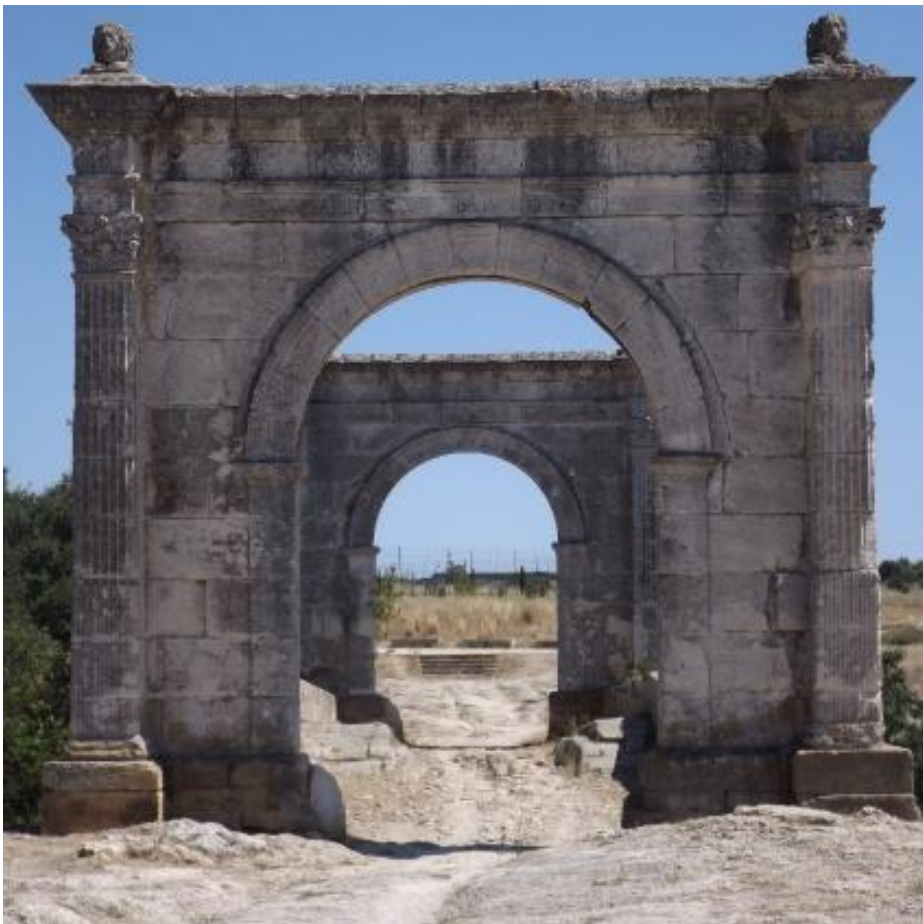
Figure 48 & 49: The Pont Flavien in Saint-Chamas in France, one of the few Roman bridges to retain both its original arches. An inscription can just be made out just above the arch. Author images.
