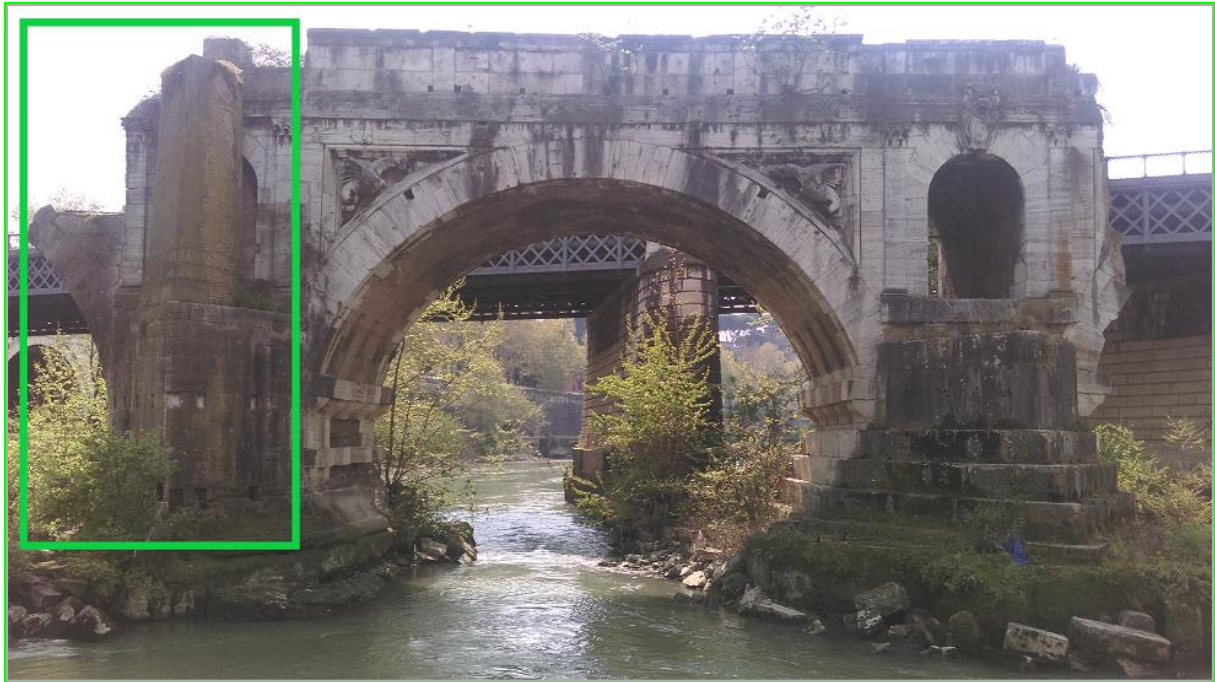
Figure 2: The remaining arch of the bridge known as the Ponte Rotto. The only ancient elements of the Pons Aemilius are part of the foundations and interior of the eastern side of the arch (within the area highlighted in green). The photo above was taken from the Tiber Island facing downriver. Image: Author.
