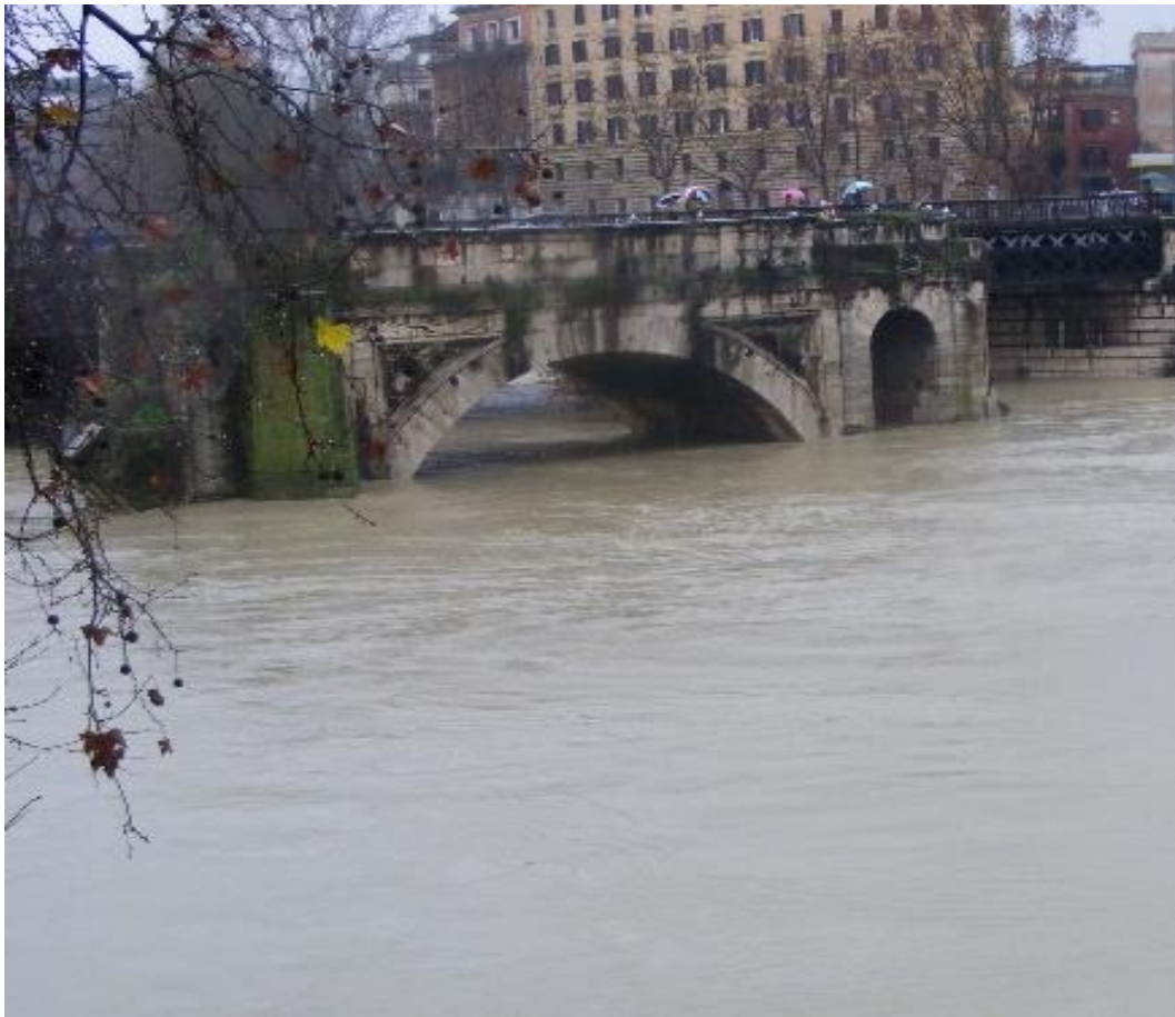
Figure 35 & 36: Pons Aemilius in the winter of 2014. The photos were taken a day apart and illustrate just how quickly the Tiber level can change, even with the modern embankments. Author image 2014.
