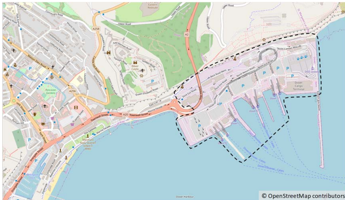
Figure 1. Aerial view of the Port of Dover Eastern Docks (Source: [26]). The black dashed line roughly marks out the physical boundary of the Eastern Docks.
