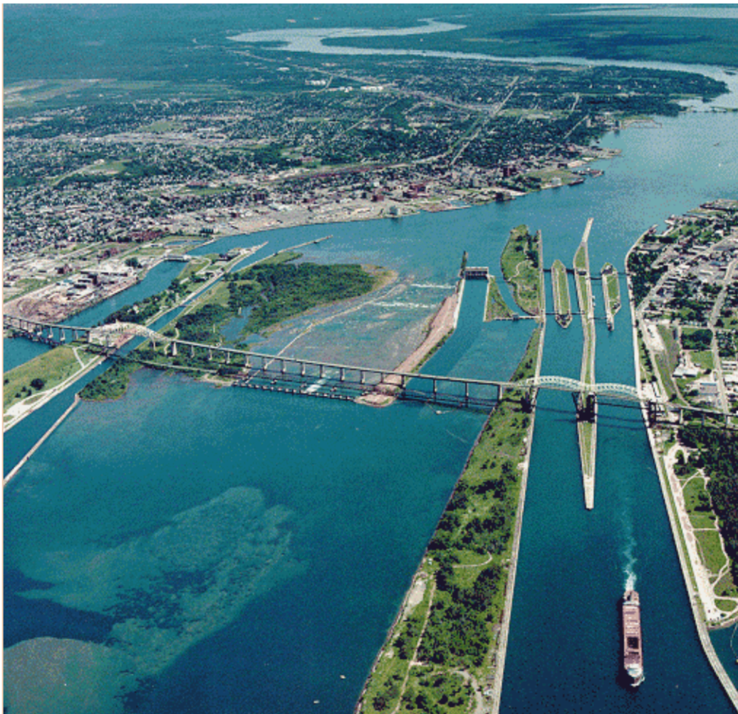
United States Army Corps of Engineers, "Aerial picture of the Soo Locks (downriver view)", United States Army Corps of Engineers (August 15, 1992)
