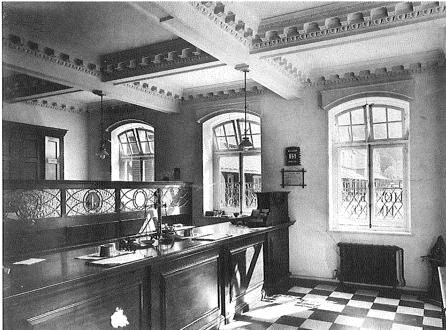
Fig. 7. Lloyds Bank, 151 London Road, Southborough, Kent (1912–14): interior view. Undated photograph, c. 1920
