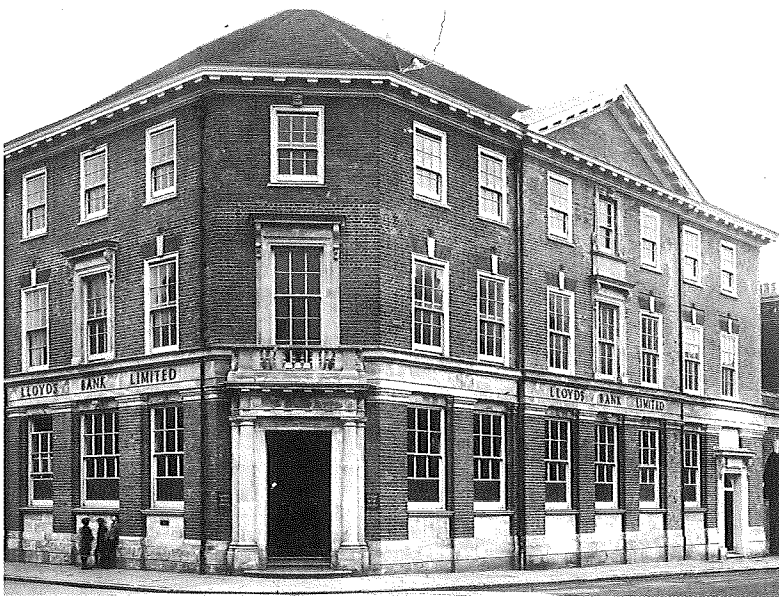
Fig. 13. Lloyds Bank, 81 High Street, Ashford, Kent (1924–25). Photograph of 1927
