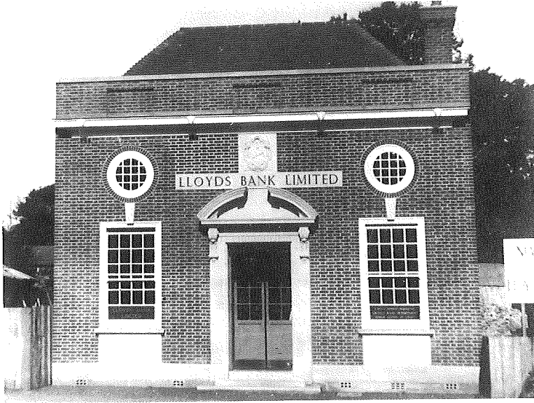
Fig. 16. Lloyds Bank, High Street, Hartley Wintney, Hampshire (1927–29). Photograph of 1929
