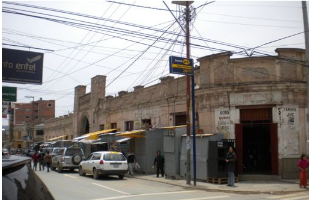
Figure 29. Western perimeter of Fermin Lopez marketplace.
