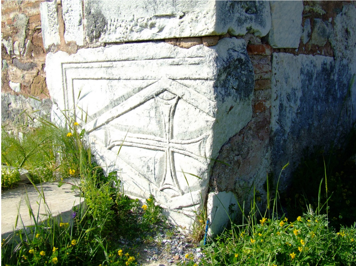
Figure 22. Cross-domed church of St. Mary: detail of reused chancel parapet incorporated in the southeast corner of the southeast pier (author's photo)
