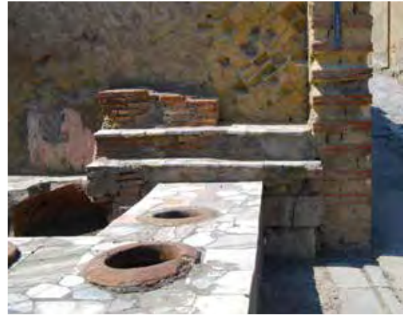
Fig. 5.41 Counter at IV.15-16 Herculaneum with stepped shelves built out towards the front of the shop.
