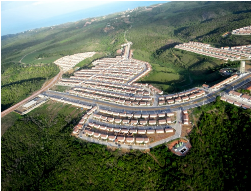
Figure 3: Maceió-AL, Minha Casa Minha Vida social housing aerial view, 2014. Photography courtesy of the Laboratory QUAPÁ, from the Faculty of Architecture and Urbanism, University of São Paulo – FAUUSP, Brazil.
