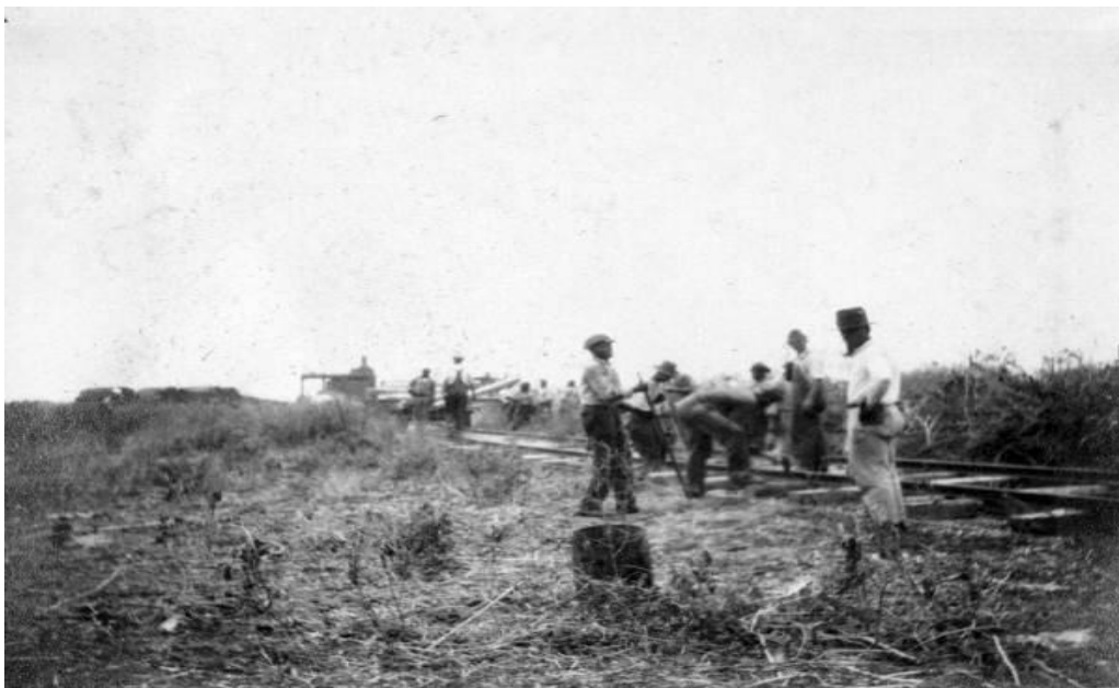
Fig. 13. Rails being spiked while building the Moore Haven and Clewiston Railway (1921)
