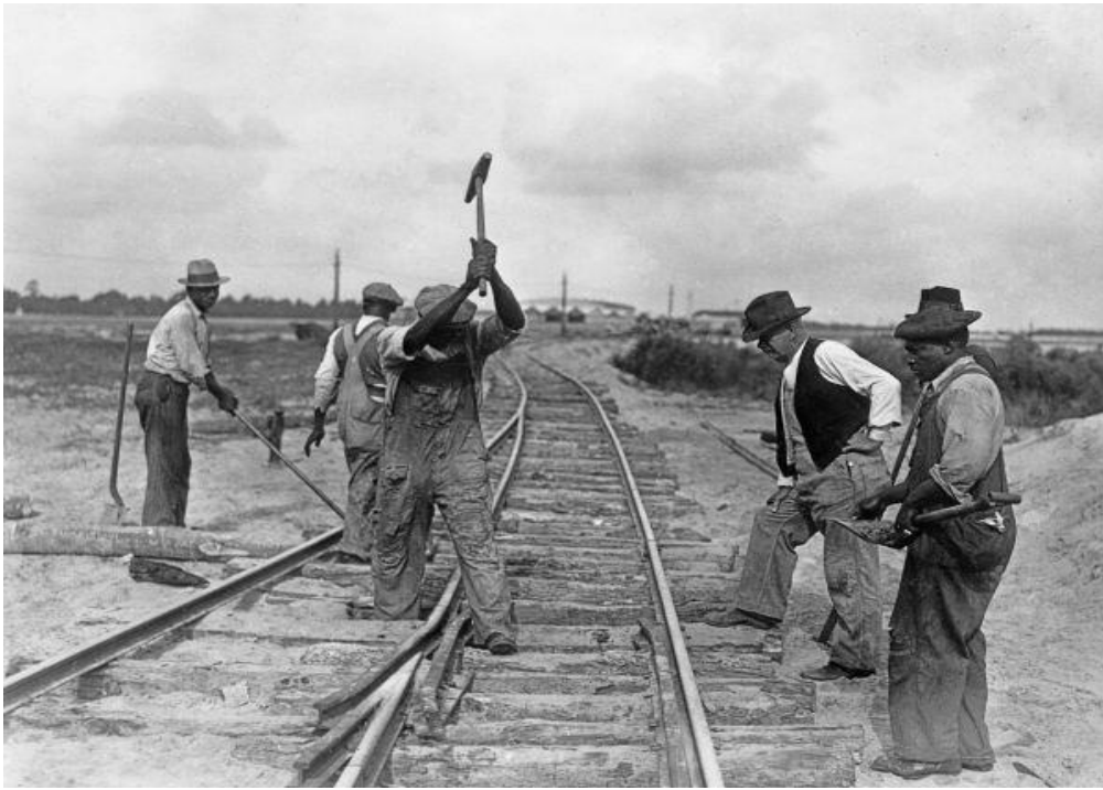
Fig. 12. Laying railroad track for airport construction in Jacksonville (1934)
