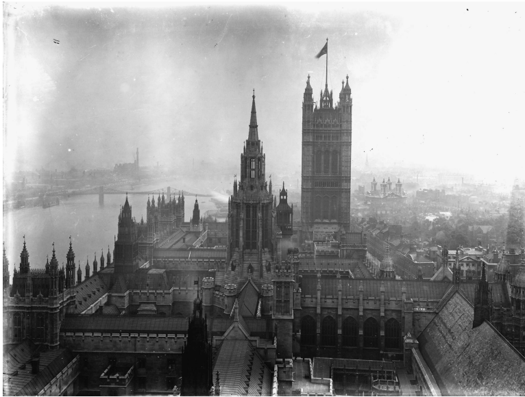
Fig 11. Aerial view of the Houses of Parliament (looking eastwards) showing the position of local ventilation shafts introduced by Reid and Barry after abandoning the central up-cast shaft in 1846, c 1900, PED: Farmer 743. Photograph: © Parliamentary Estates Directorate.
