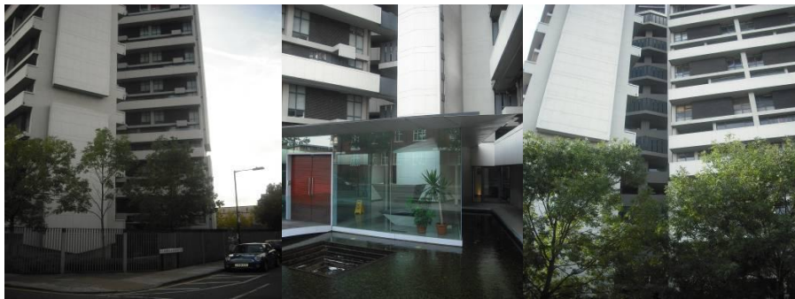
Figure A1.8: External views of Keeling House, Clerdale Street in Bethnal Green, London showing clustered arrangement of apartments with centrally placed water body in the foyer at the ground floor which can possibly improve the thermal conditions of the building in summertime.
