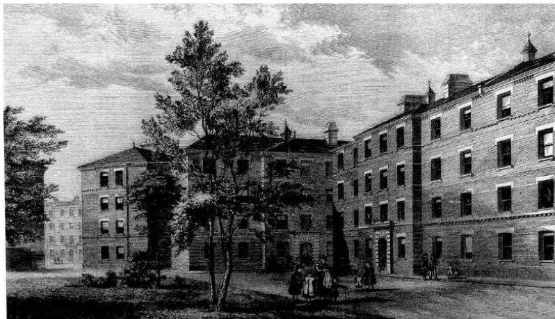
Figure A1.2: External view of the Peabody Square housing development in London (1880s), a good example of philanthropic housing provision showing decorative cornice along the facade clad in bricks, large openings for natural ventilation and lighting and hip-gable roof with projecting chimney used for heating (Campbell, 2008).
