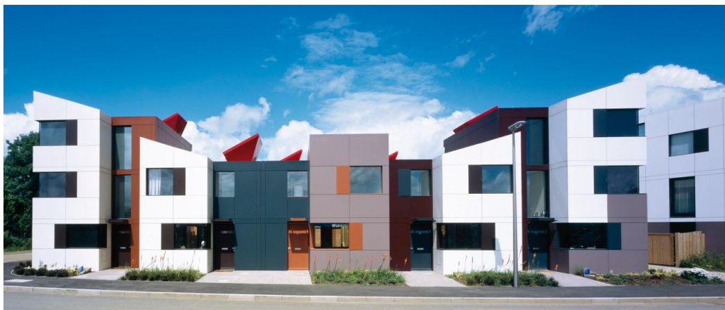
Figure 5.15: Different views of the overall skyline of urban scene at Oxley Park with the Eco-Hat placed on the roof of each house to improve energy efficiency of the development (RSHP, 2008).
