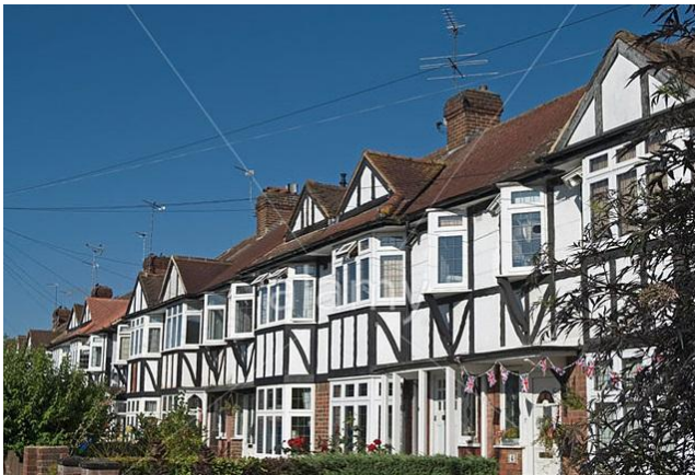
Figure A1.6: Mock-Tudor housing development built during the interwar period in Ham, Surrey showing a typical arrangement of houses with replicated style and decorative timber, striking gable and the houses are clad with less stylish timber and provision for minimum setback as specified in the space standards and rear private gardens (Alamy, 2014).
