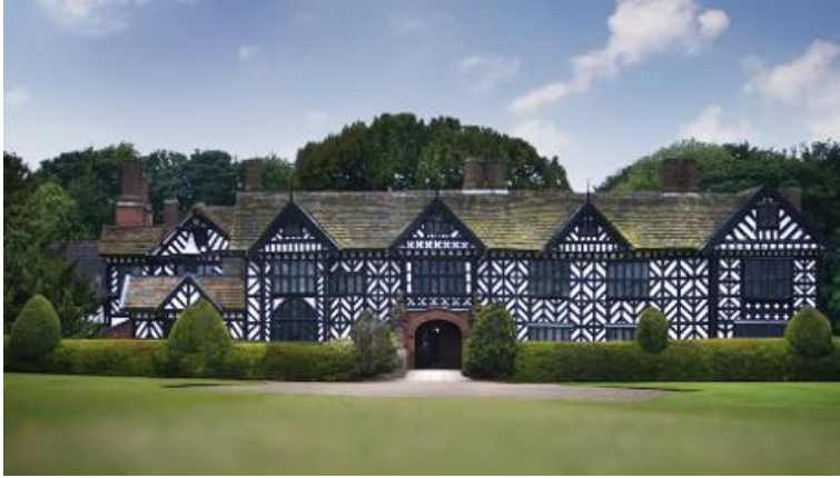
Figure A1.3: View of a Mock-Tudor manor house located at the banks of the River Mersey in Liverpool built in the 19th century showing the ornamented facade with a unique black and white timber materials suggesting a blend of Victorian architecture with features of traditional Tudor timber-framed construction and crafts covered with slates material laid on striking gable roof (National Trust, 2013).
