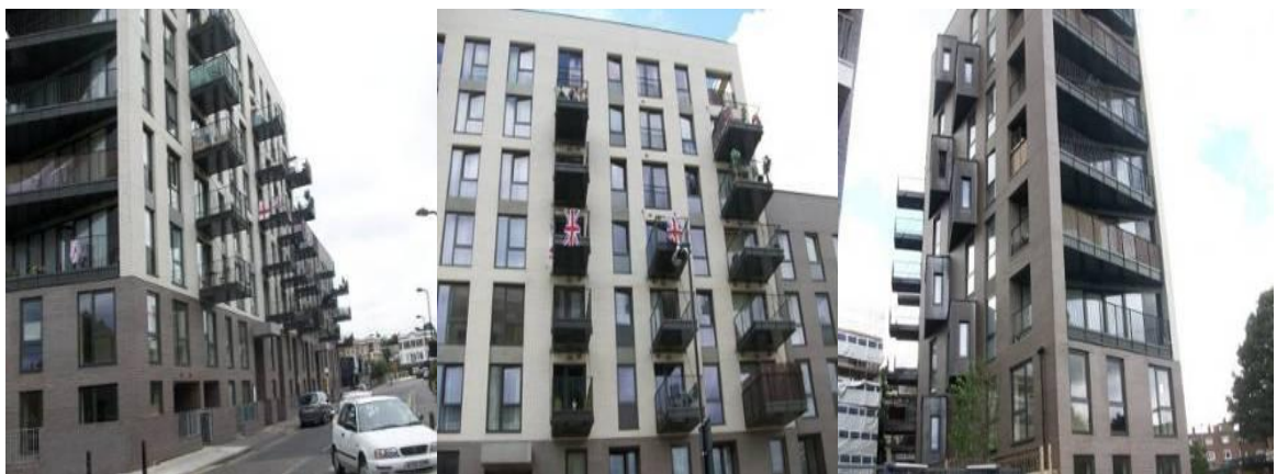
Fig. 5.10: Different views of Bridport House showing high-quality brown bricks outlining the height of the maisonettes from the upper floors at the 8-storey block and demarcating the 5-storey block of apartments.
