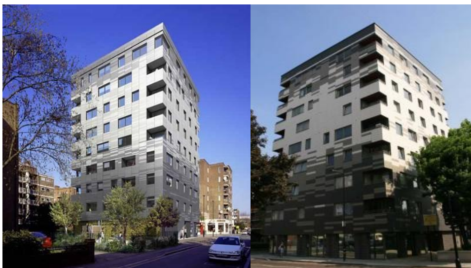
Figure 5.21: Street views of Stadthaus in Murray Grove, London showing a strong connection with the environment (Thompson, 2009).
