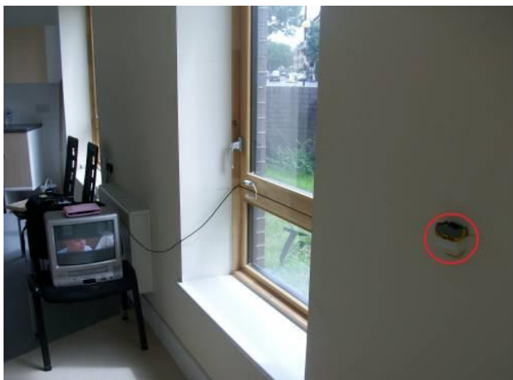
Figure 4.3: View of FL1GFL at Bridport showing the data logger in red circle mounted on the internal wall at the height of 1.1m above the floor level during the summer survey.
