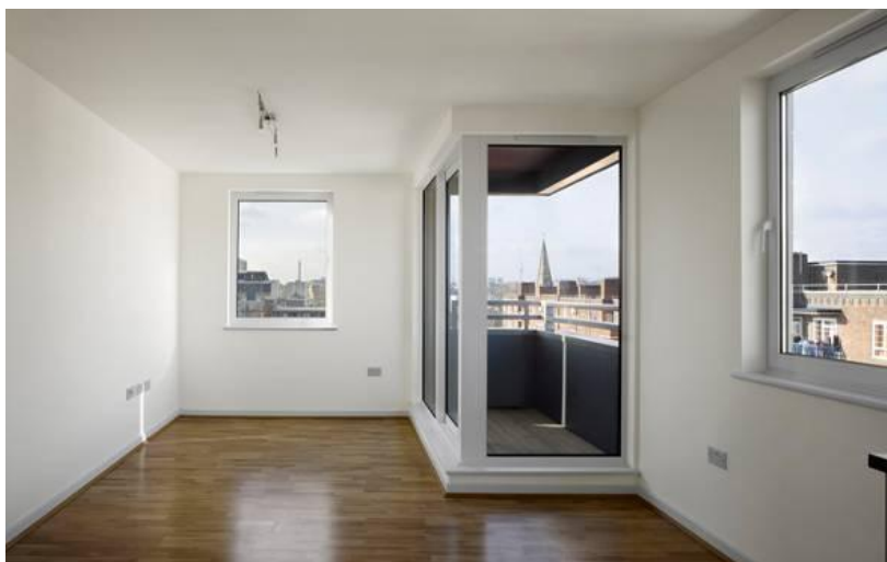
Figure 5.24: Interior walls of Stadthaus covered with plasterboards to give the indoor environment a false impression of apartments built with conventional building materials (Thompson, 2009).
