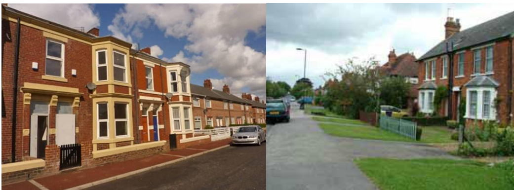
Figure A1.5: External view of ‘Byker’ flats in terraced housing in one of UK cities (Newcastle- left) and Edwardian suburban housing in Maidenhead (right) with centrally positioned openings over decorated entrance areas with left entrance leading directly to the first floor flat while the right entrance leads to the ground floor flats.
