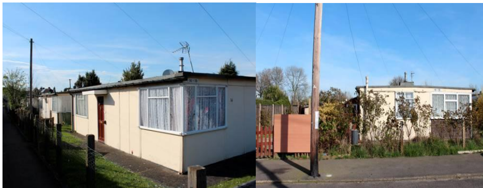
Figure A1.7: Views of the Excalibur Estate in London, a timber-framed post-war speculative mass-produced housing development showing timber flat roofs, corner windows and paneled plywood doors (Prefab Museum 2014).
