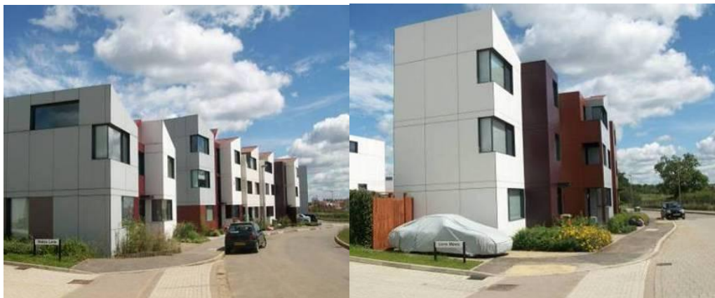
Figure 5.14: Views showing arrangement of the prototypes- Types A, B and G (left) and social housing- Types I-J adding a striking feature to the overall skyline of urban scene at Oxley Park.
