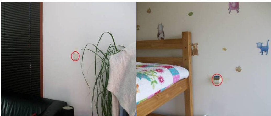
Figure 4.7: Internal views of A1WLGFL in A1WL (left) and A6MLSFB in A6ML (right) at Oxley Woods showing the position of the sensors in red circle mounted on the walls during the surveys.
