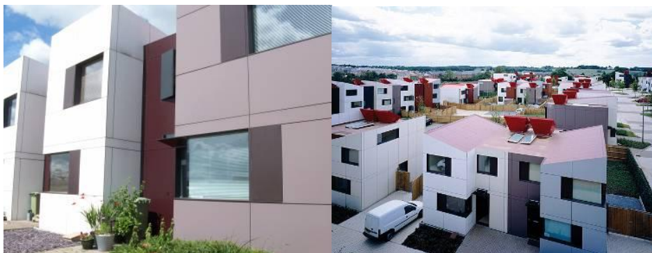
Figure 5.17: Arrangement of the cladding material (Trespan) made in different colours to provide visual expression with striking features (left) and an aerial view of the houses at Oxley Woods. (Fig 5.17b by RSHP Architects)
