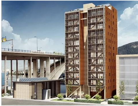
Figure 3.5: View of the 14-storey (49m high) timber tower block of 62 apartments built with CLT and Glued laminated timber (Glulam) materials in Bergen, Norway to be completed in October, 2015 (CIOB, 2014).
