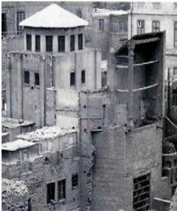
Figure 3-10: Malkaf in the house of Moheb El Deen - Cairo - fifteenth century (Steele 1997).
