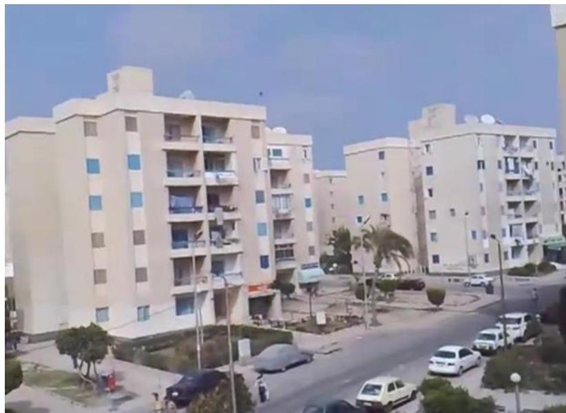
Figure 7-13: The housing project photo.
