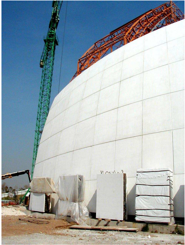
Figure 4. The smaller shell after its completion. At its bottom some ashlar ready to be assembled for the medium-size shell. (Picture by the author, taken 04/04/2001).
