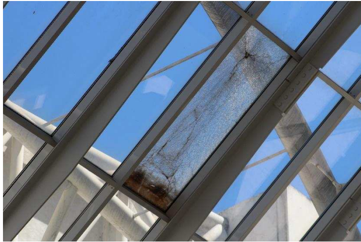
Figure 17. A broken glass panel of the roof. truss (Picture by the author, taken 22/05/2016).
