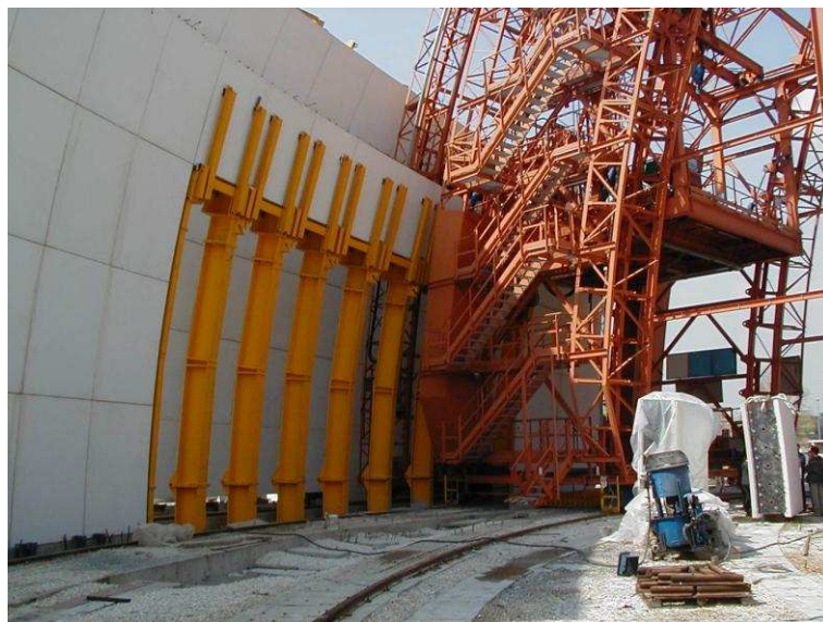
48 49 Figure 3. The travelling crane built to assemble the ashlar of the three shell. (Picture by the author, taken 50 04/04/2001). 51 52 53 54 55 56 57 58 59 60 61 62 63 64 65
