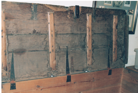
Fig. 16 'Bites' showing two of original four positions of mortised knuckle hinges, Faversham.
