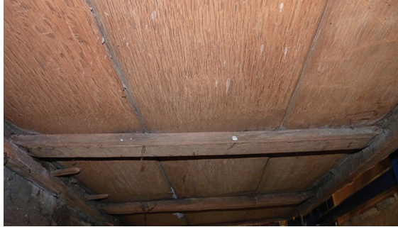
Fig. 13 View underneath showing supporting battens and pegs fixing apron, Norwich.
