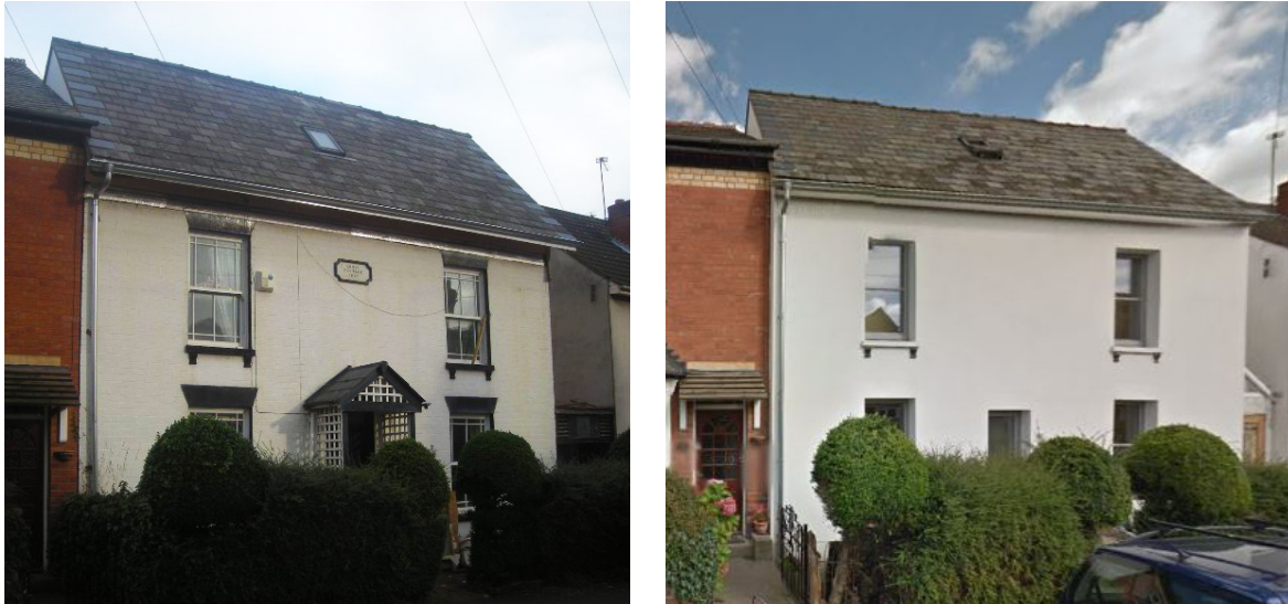
Figure 05 : Pre-retrofit and post-retrofit images illustrating the approach to the facade (Low Energy Building Database, 2010)
