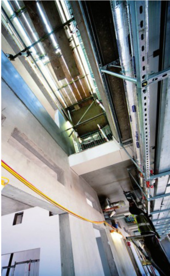
Figure 16: Interior construction photograph
