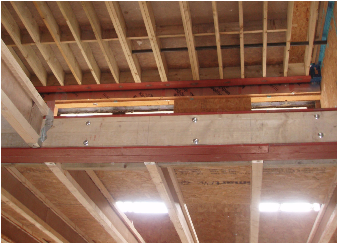
Figure 31 : Working construction photograph displaying the new steel beam and timber joists
