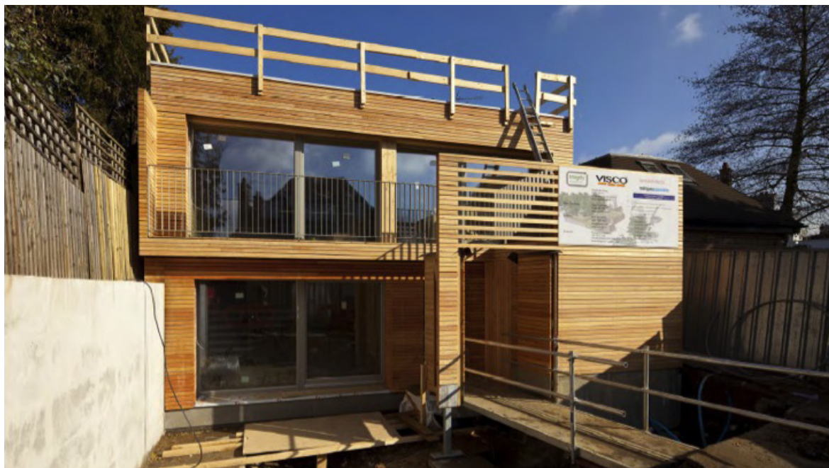
Figure 14 : Exterior View of Last Stage Construction (Bere:architects, 2010)
