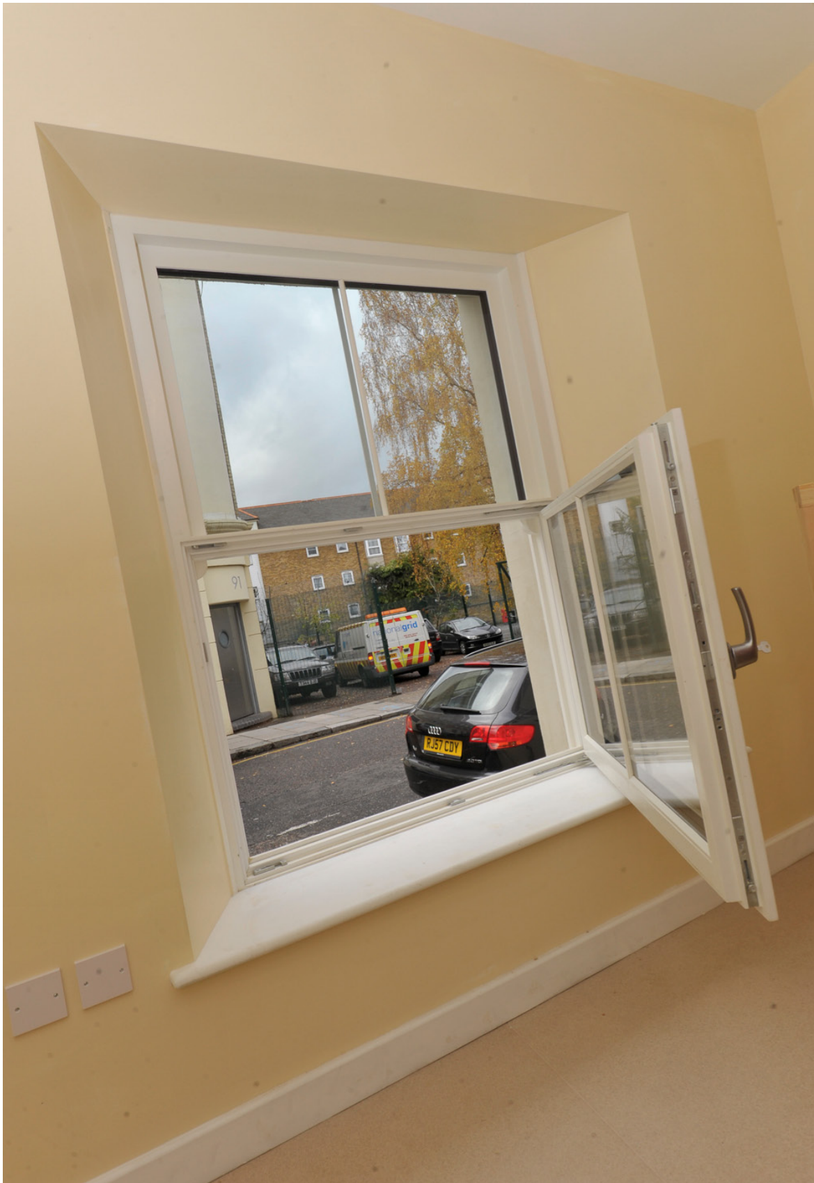
Figure 22 : The new mock sash windows with a side hung bottom casement and fixed upper pane
