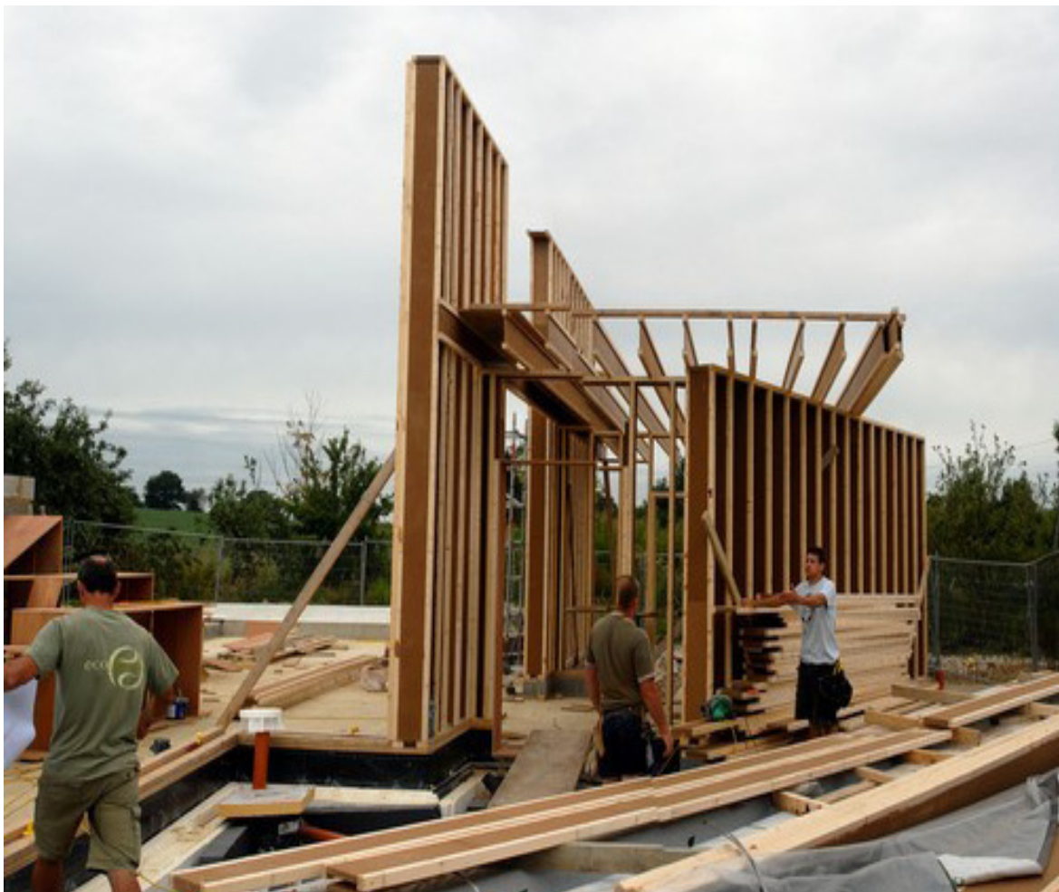
Figure 06 : Steico Timber Frame being constructed
