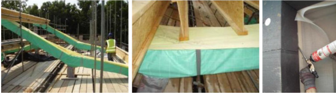
Figure 14 : Centre for Disability Studies - airtightness of walls and roof.
