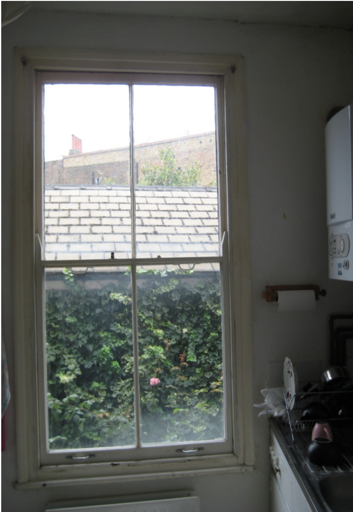
Figure 21 : The existing sliding sash windows of 100 Princedale Road, before works began
