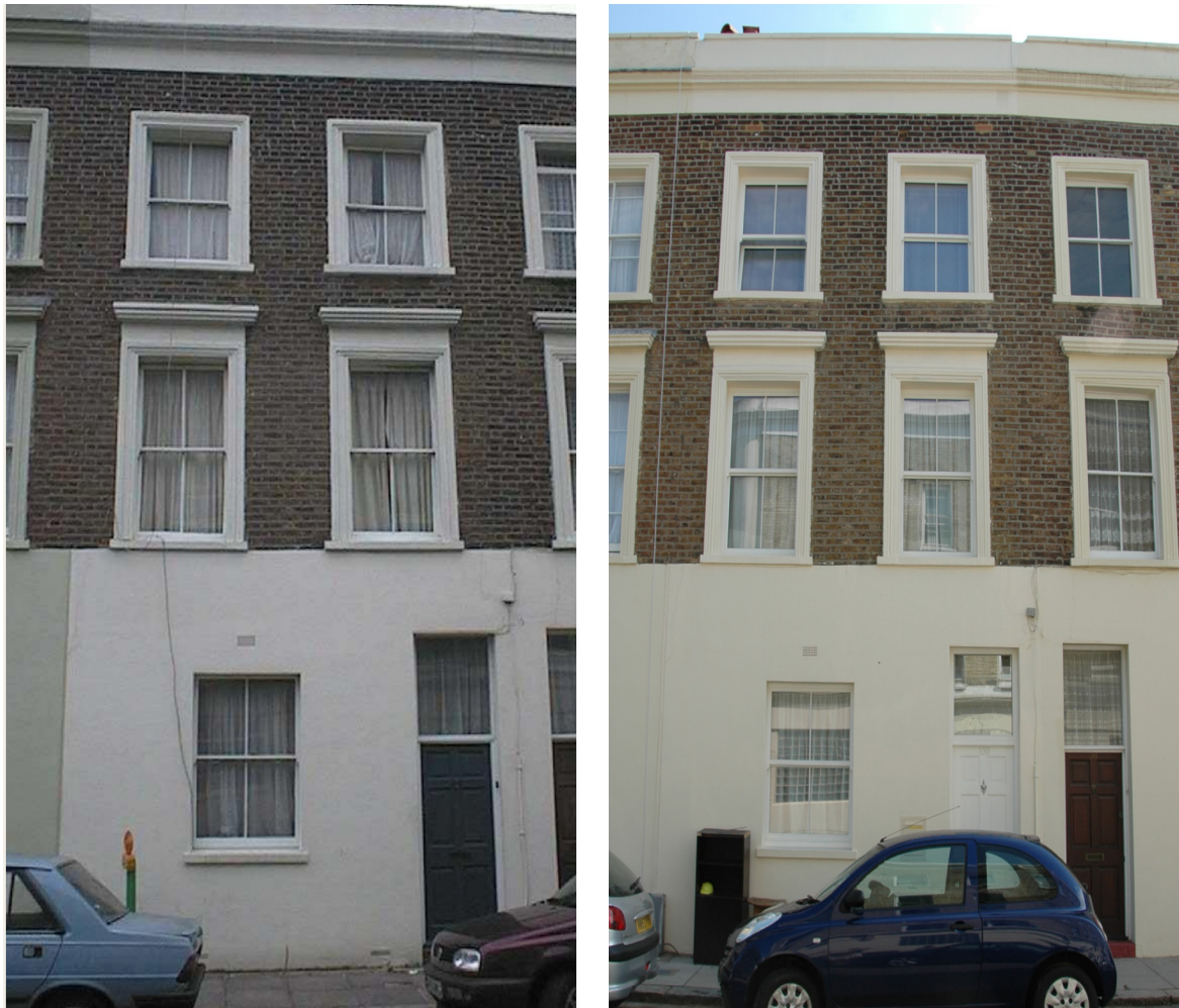
Figure 20 : Before and after front elevation photographs of 100 Princedale Road.
