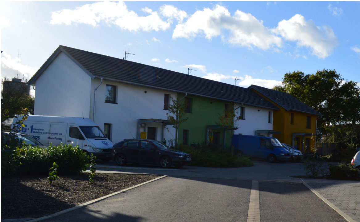
Figure 03: Wimbish Passivhaus units 7-10 (Own Photograph)
