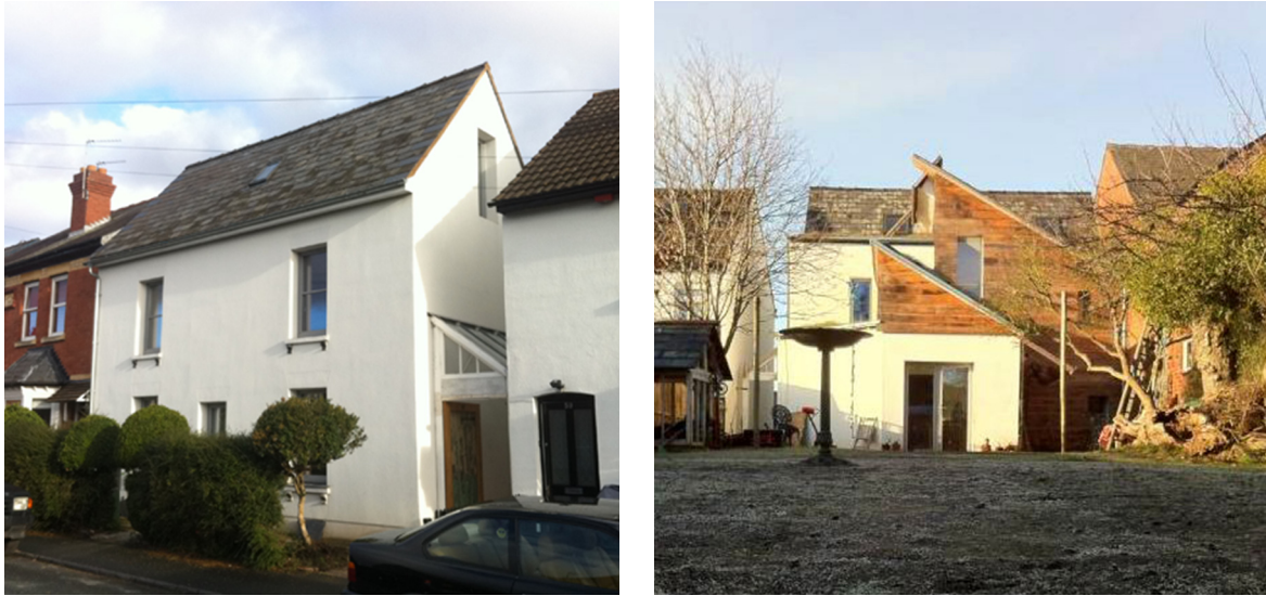
Figure 01: Post-retrofit illustrating externally insulated existing building and new-build extension (Low Energy Datatbase, 2010)
