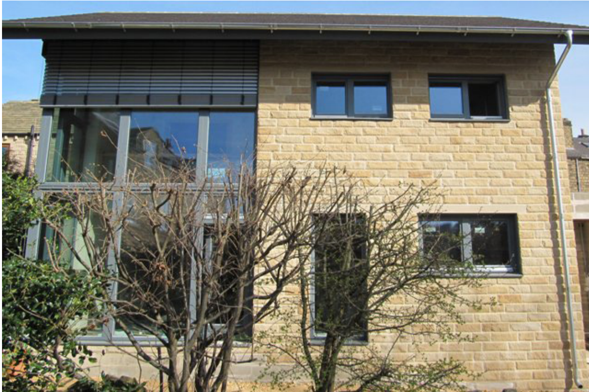
Figure 03: Denby Dale external facade
