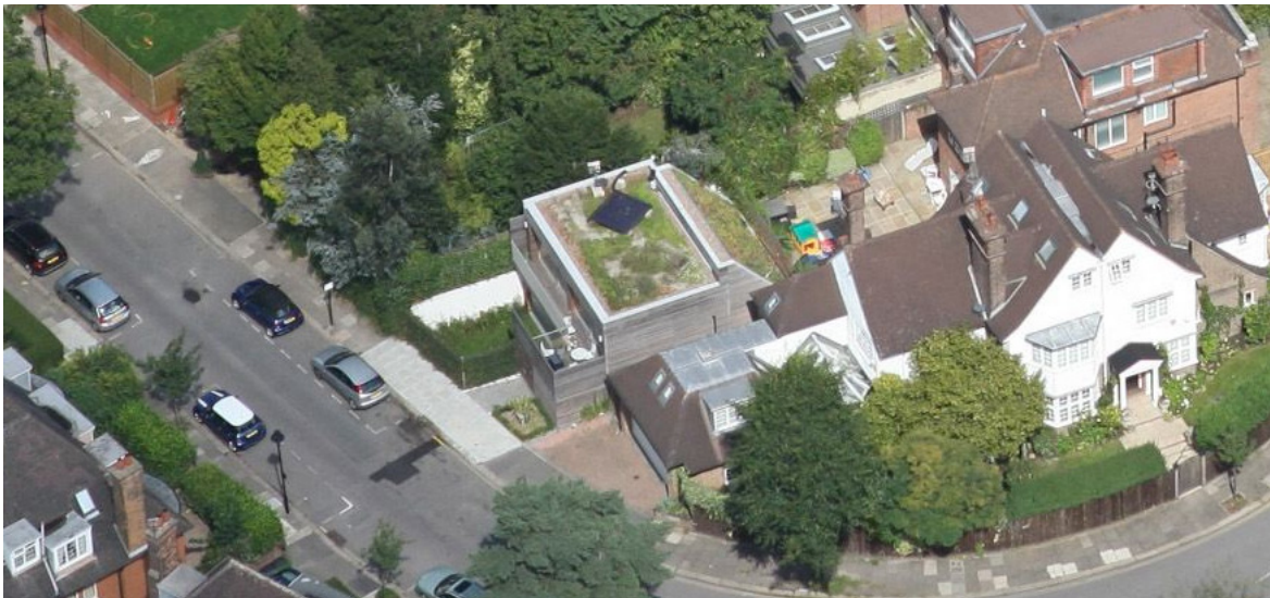
Figure 01 : Aerial View - Camden Passivhaus (Bing Maps, 2013)
