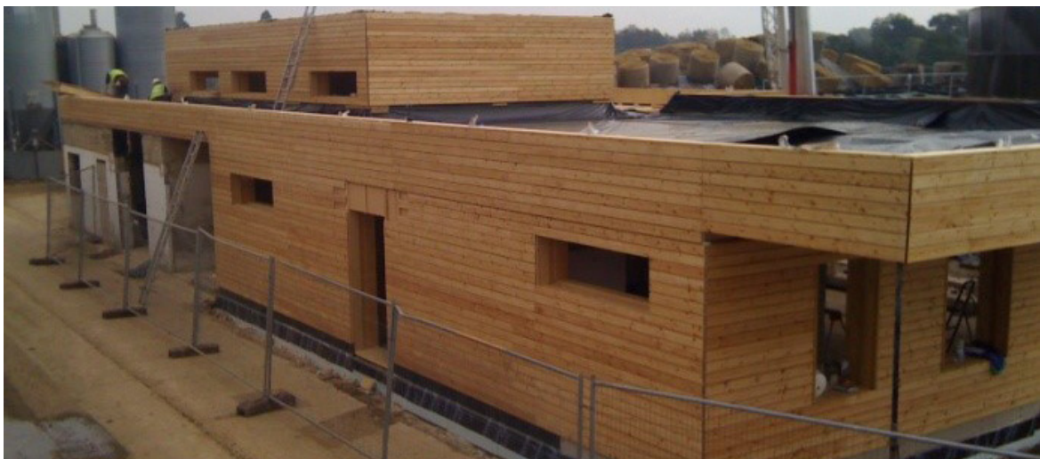
Figure 11 : Day 3 of panel installation
