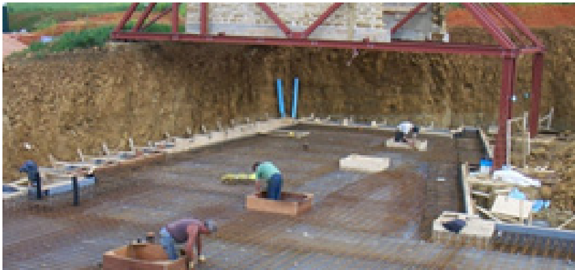
Figures 05: In-situ concrete poured over insulation, waterproofing & reinforcement bars.
