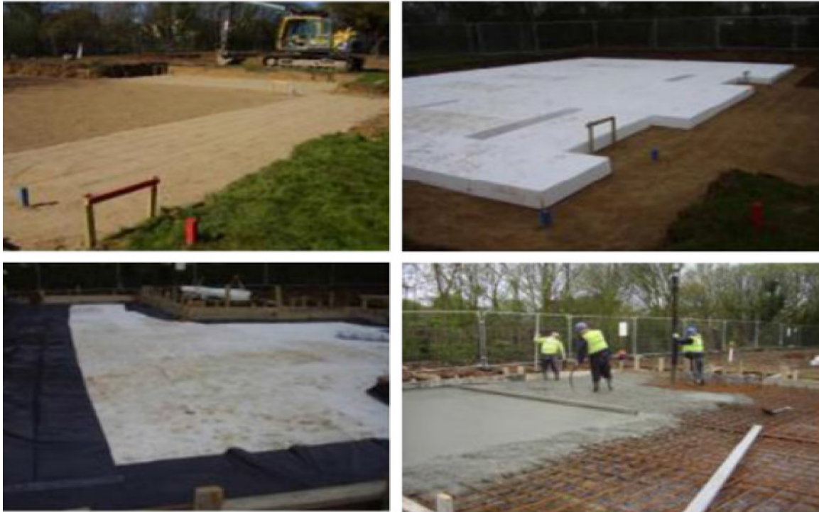
Figure 09 : Floating foundation system under construction.
