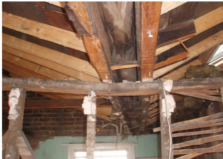
Figure 7 : Internal view of the existing butterfly roof structure - 100 Princedale Road
