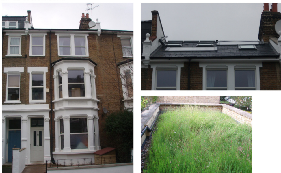
Figure 25 : Completed photographs of the Passivhaus retrofit at Lena Gardens, London
