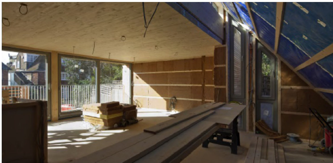
Figure 13 : Interior Construction Works (Bere:architects, 2010)
