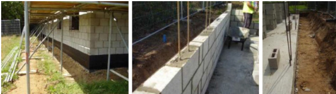
Figure 15 : Centre for Disability Studies - airtightness of foundation and ground floor.
