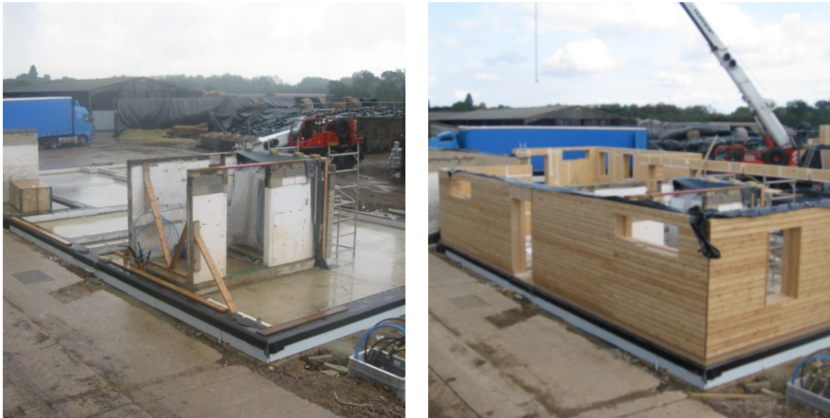
Figure 09 & 10 : Day 1 and Day 2 of panel installation
