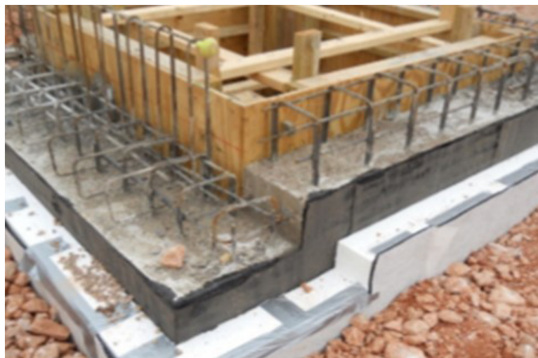
Figure 10: Photograph showing the construction process.
