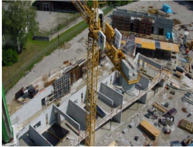
Figure 14: Photograph showing the German Passivhaus School using a concrete panelled method of construction.
