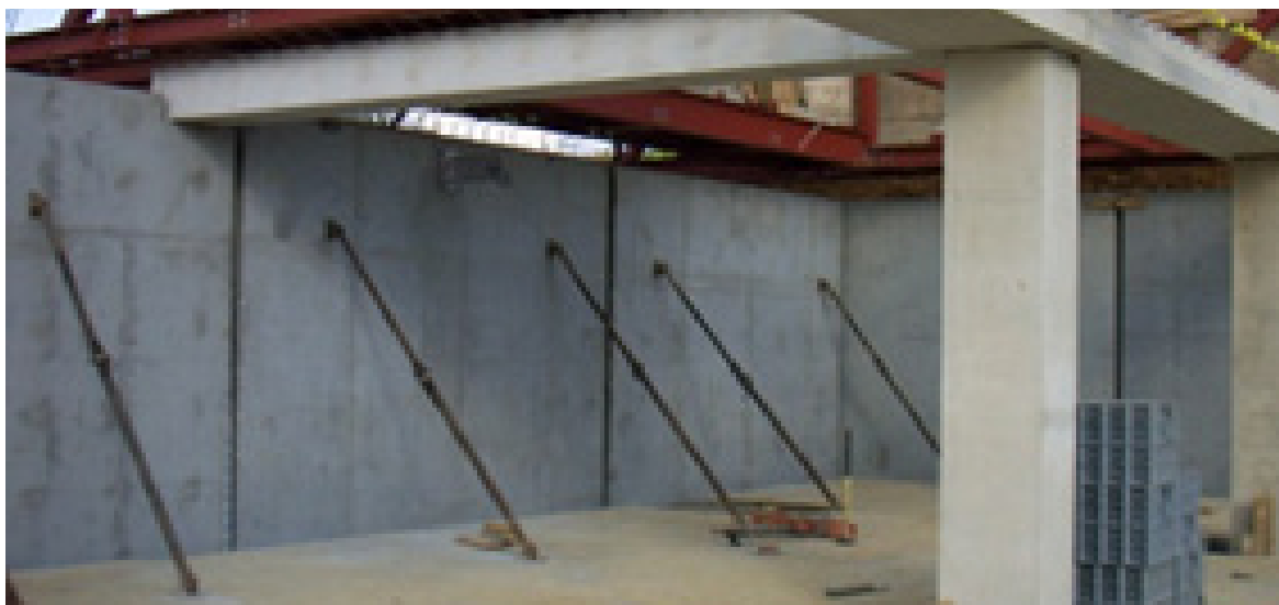
Figures 06: Precast concrete panels of Underhill House.
