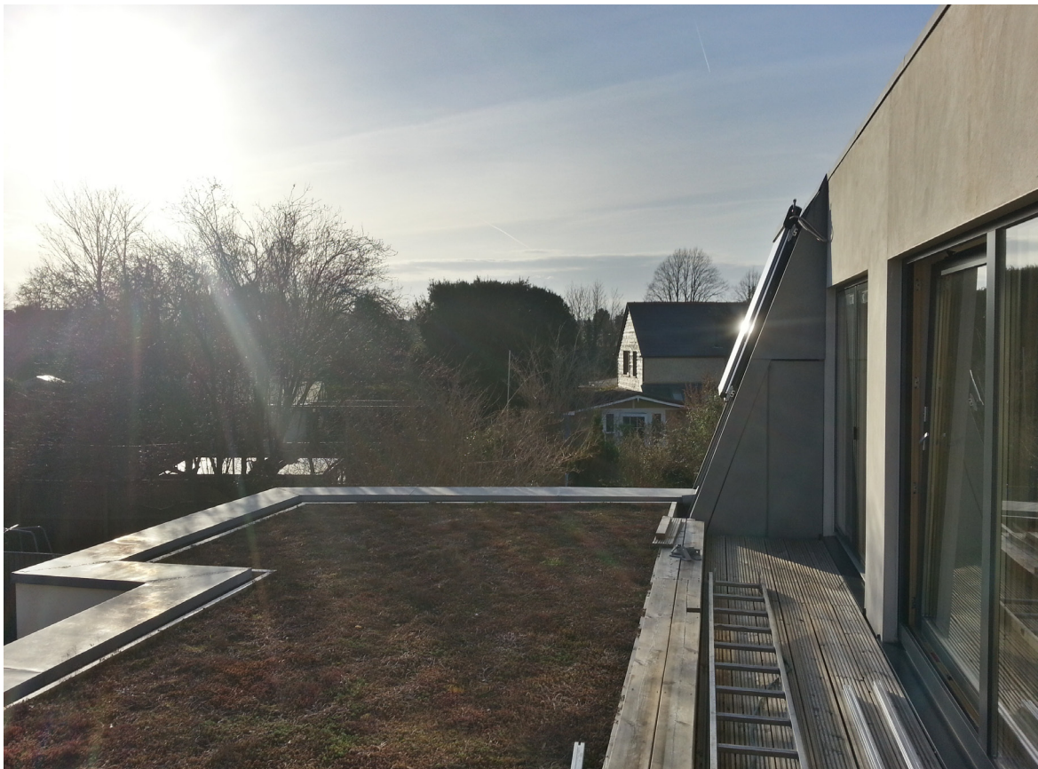
Figure 9: Green Roof and solar panel
