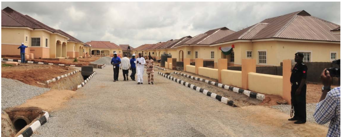
Figure 2.2: Typical lower-middle income housing estate in Abuja Nigeria, Source: Google/images
