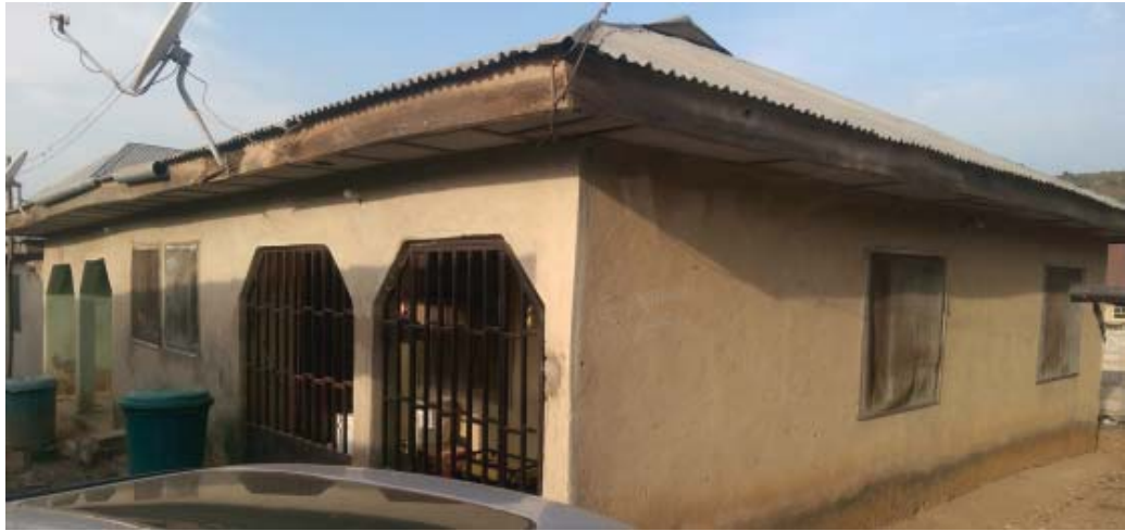
Figure 4.38: BWH1NV at Bwari, Abuja, showing the main building.
