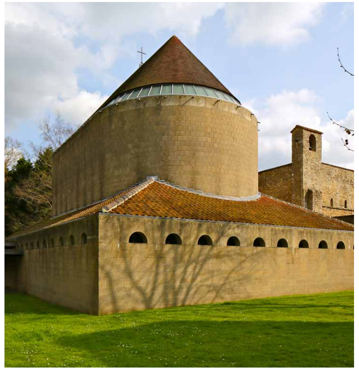
Fig 11. View from the north-west of the new Abbey Church at West Malling, Kent, designed by Robert Maguire and Keith Murray, 1962-6. The community moved to the vicinity of the ruins of the old church (currently used as chapter house), visible in the background, in 1916. Convent building listed Grade I; refectory Grade II; church is not listed.
