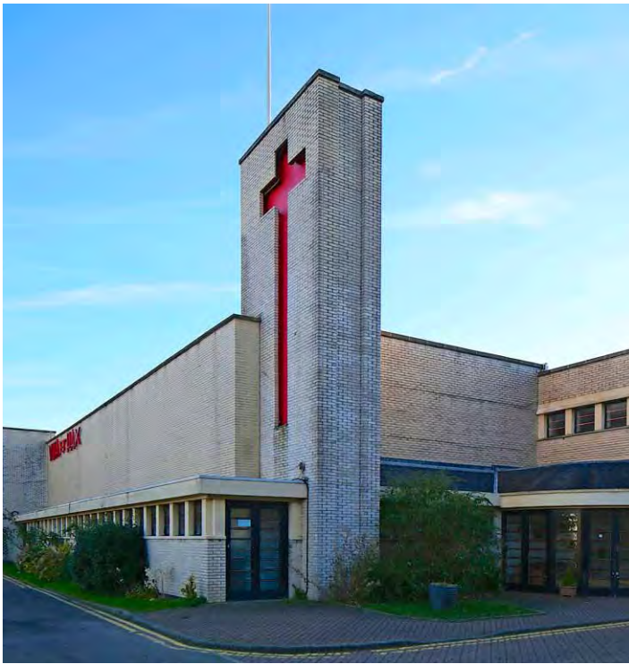
Fig 10. The monastery of the Olivetan Benedictines at Cockfosters, on the far northern fringes of London, was designed by Dom Constantine Bosschaerts. Although built in 1940 in a form that was much reduced from that originally proposed, the building is remarkable for its Dutch Expressionist style, more associated with cinema architecture.
