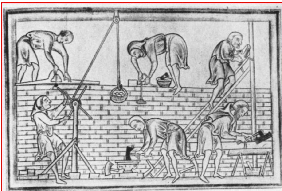
Fig. 1. Thirteenth Century. Reproduced from L. F. Salzman, Building in England down to 1540 , by permission of the Clarendon Press, Oxford.
