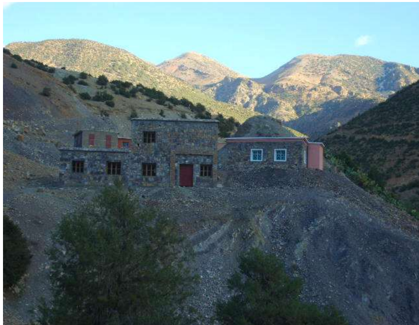
Plate 9.9: View of completed distillation building (El Maghzen, November 2008).
