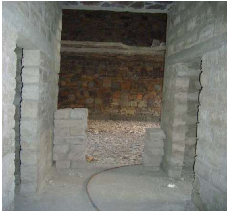
Plate 9.8: A view from the laboratory of the unfinished main room where the alembic will be installed (El Maghzen, May 2008).
