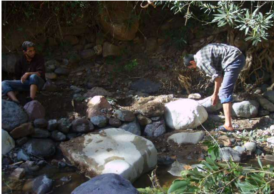
Plate 7.21: Dam building (El Maghzen, July 2008).
