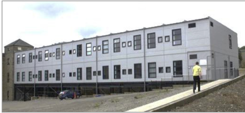
Fig. 2. The East facing façade of the 2008 modular building at Bradford Royal Infirmary.
