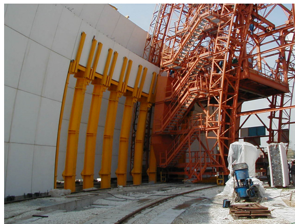
Fig. 3 The travelling crane built to assemble the ashlar of the three shell. (Picture by the author, taken 04/04/2001).
