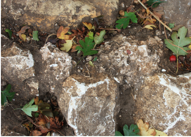
Figure 5.6 Trench J. Mortar in situ in the western wall of Building 2.
