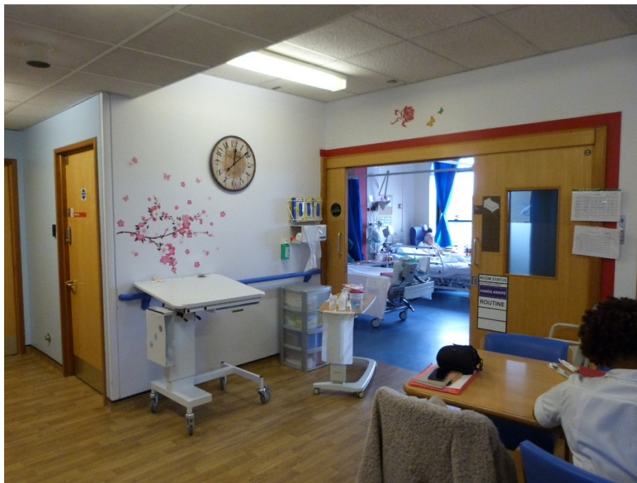
Figure 4 - An entrance to a bed-bay with color coded frame that lacks impact as it is not distinguishable from the surrounding decor
