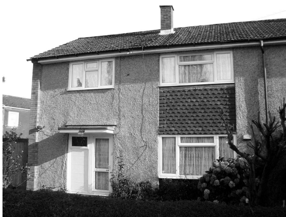
Figure 2: The Nine Acres house, constructed in 1950's using the Wimpey no-fines method
