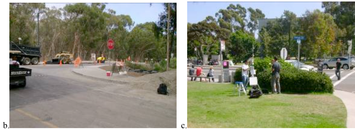
Fig. 1: (a) Overview of the survey sites (adapted from Google Earth), (b) Gilman shuttle stop TS with the DEMROES station visible in the centre, (c) Construction site CS.
