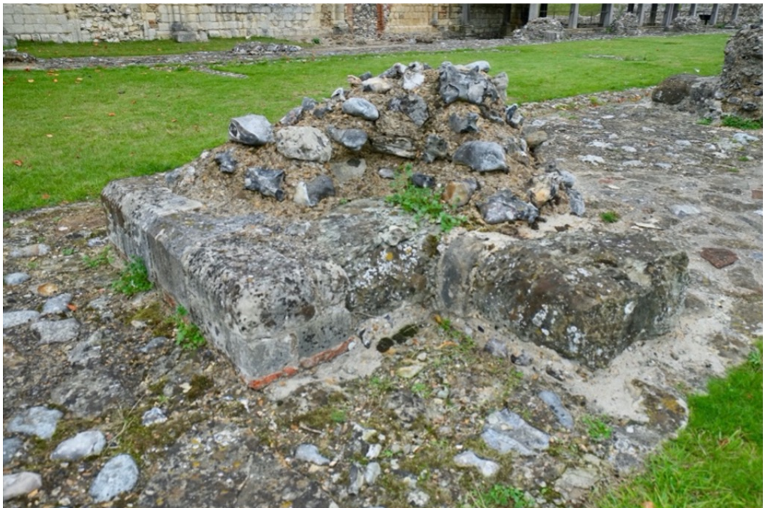
Figure 3.6: Ruin of third Norman column from east to west at the nave area, St Augustine's Abbey, Canterbury
