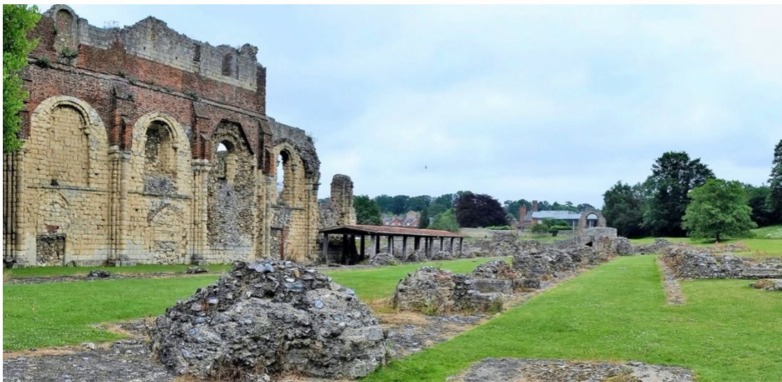
Figure 3.2: Remaining foundations of the Nave area at St Augustine’s Abbey, Canterbury
