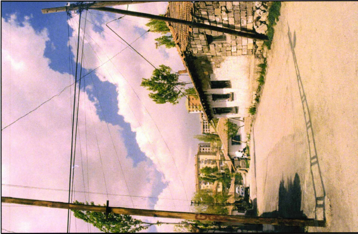
Plate D.B.1 The formal/informal divide: a view of the housing co-operative housing
