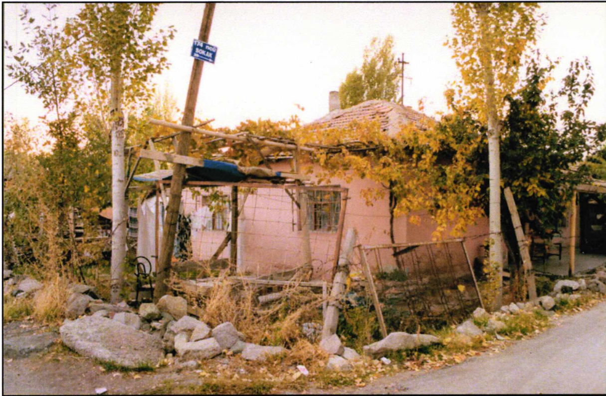
Plate D.C.1 Fencing the de facto boundaries of a Northern Ege gecekondu
