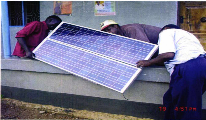
Installing a PV system at Ngasamo dispensary in Magu District (UNDP)
