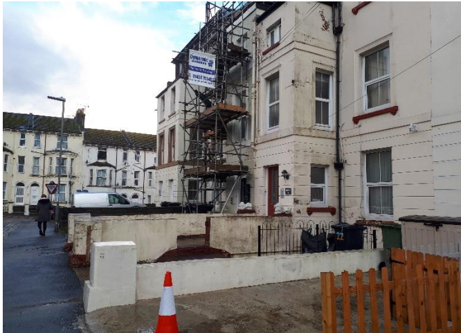
Photo 4: One of the many houses under renovation
