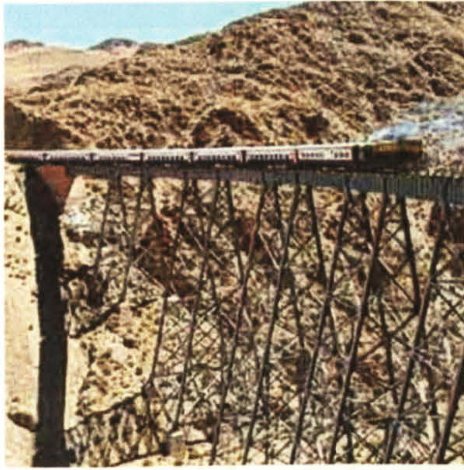
Figure 39. 1887, Train bridge, Salta
