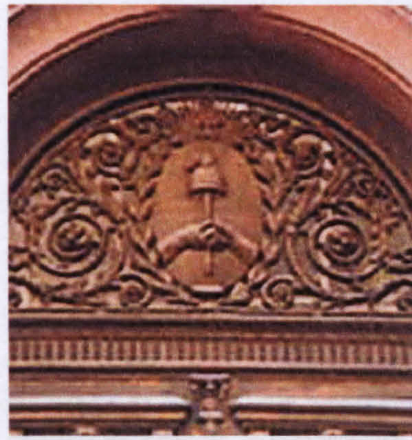
Figure 82. 1912, General Archive's building
