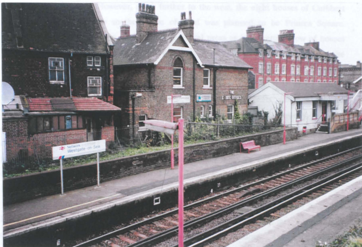
PLATE 30. Westgate on Sea Railway Station erected 1871 received complaints that it was not good enough for 'blue-blooded Westgate'.
