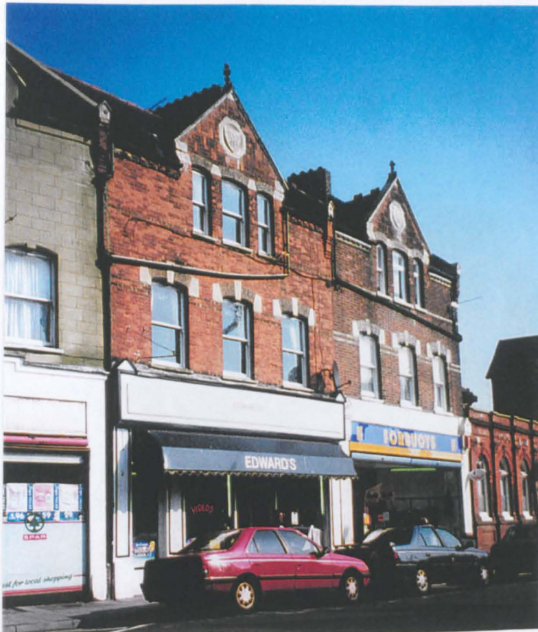
PLATES 55. Diapered brick gable with 1883 cartouche on shops at the western end of Station Road.
