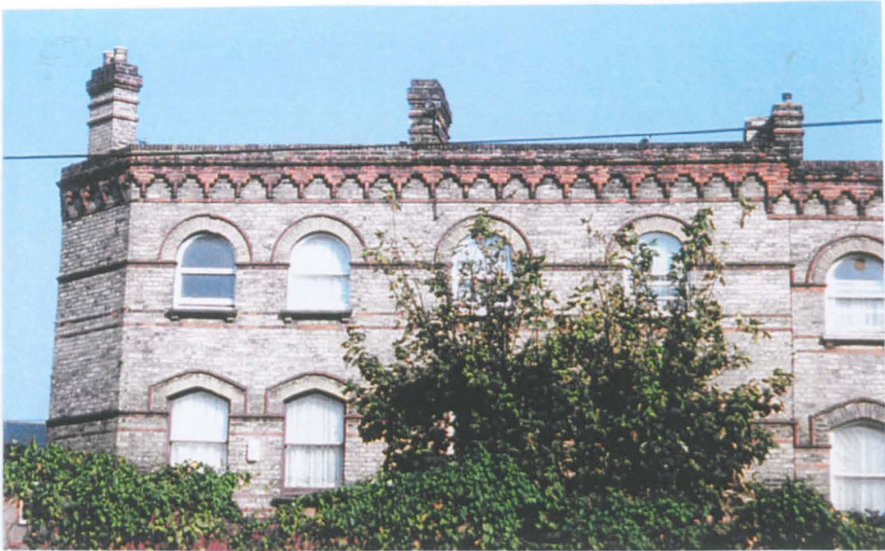
PLATE 54. High quality brickwork on the early shops at the eastern end of Station Road.
