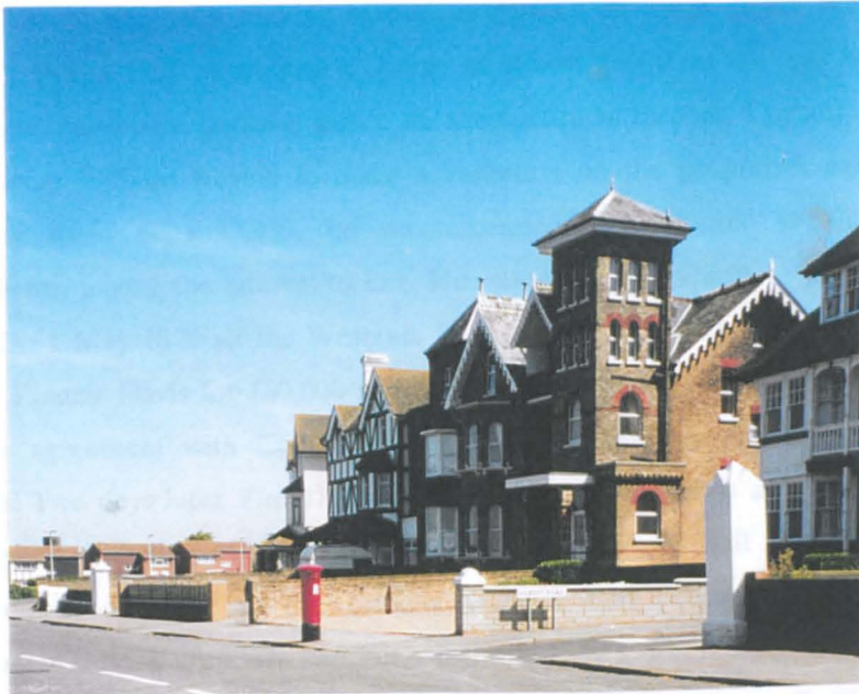
PLATE 7. Osborne House built by William Wigmore of Walham Green. Advertised in Keble's Gazette July 1875 for sale by auction. Drawing-Room 16ft by 24ft, dining-room 18ft by 16ft, library with folding doors connecting to the dining-room. Seven bedrooms, smoking room on second floor, croquet lawn. Became first County Club for Gentlemen, then successively a private residence, a girls' school and an hotel.
