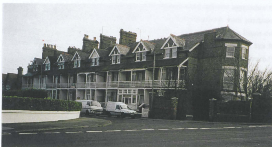
Plate 6. 1-8 Cuthbert Terrace built by Smith and Swain of Margate 1871/2. They are not shown in the 1871 census return for Minster, but are shown on Maps 3 & 4.
