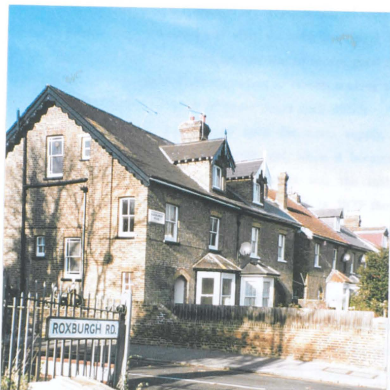
Plate 5. Semi-detached villas in Roxburgh Road west . Two were occupied by the time of the 1871 census, No. 1 by Archibald Roxburgh himself. The fourteen were completed in 1872.
