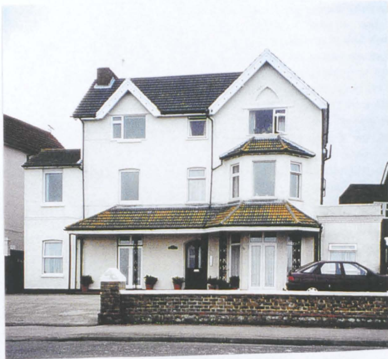
Plate 4. No. 2 Sea Road is of the same date. In correspondence of 1871, Corbett is seen to be trying to sell it. Named Cleveland's it was occupied by solicitor Henry Houseman for many years. Later it became the Northcott Guest House.
