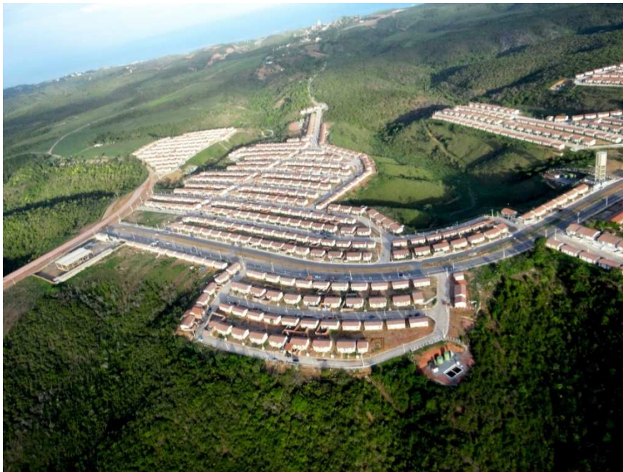
Figure 3: Maceió-AL, Minha Casa Minha Vida social housing aerial view, 2014. Photography courtesy of the Laboratory QUAPÁ, from the Faculty of Architecture and Urbanism, University of São Paulo – FAUUSP, Brazil.
