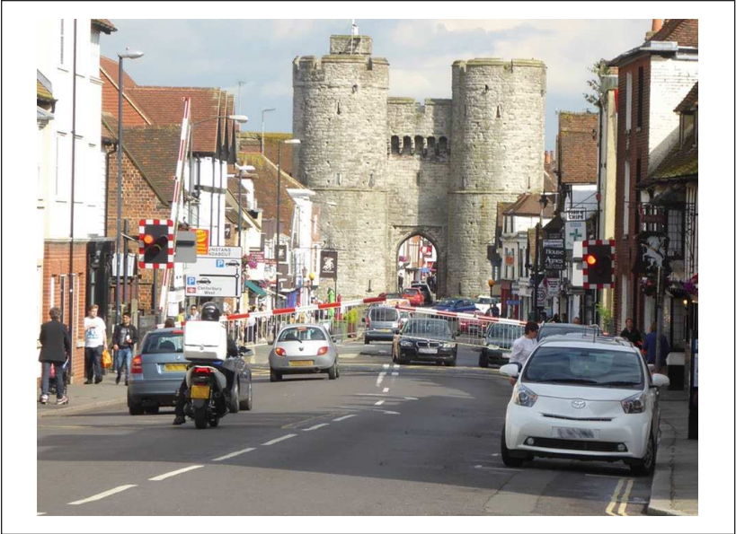
Figure 1. The level crossing and surrounding area.
