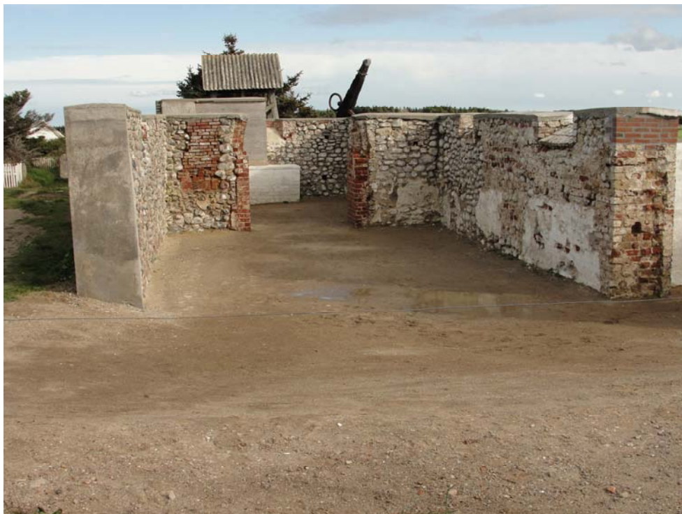
Figure 4. Mårup Church after its “creative dismantling” in 2007.
