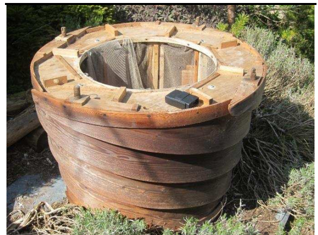
Fig 3: The air inlet terminal above the manhole
