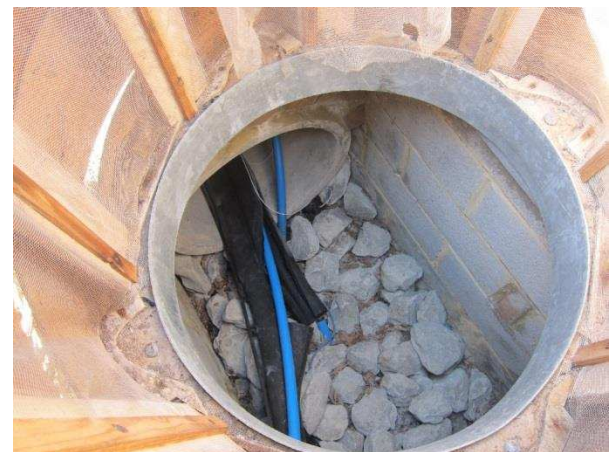
Fig 4: Junction of manhole and earth tube
