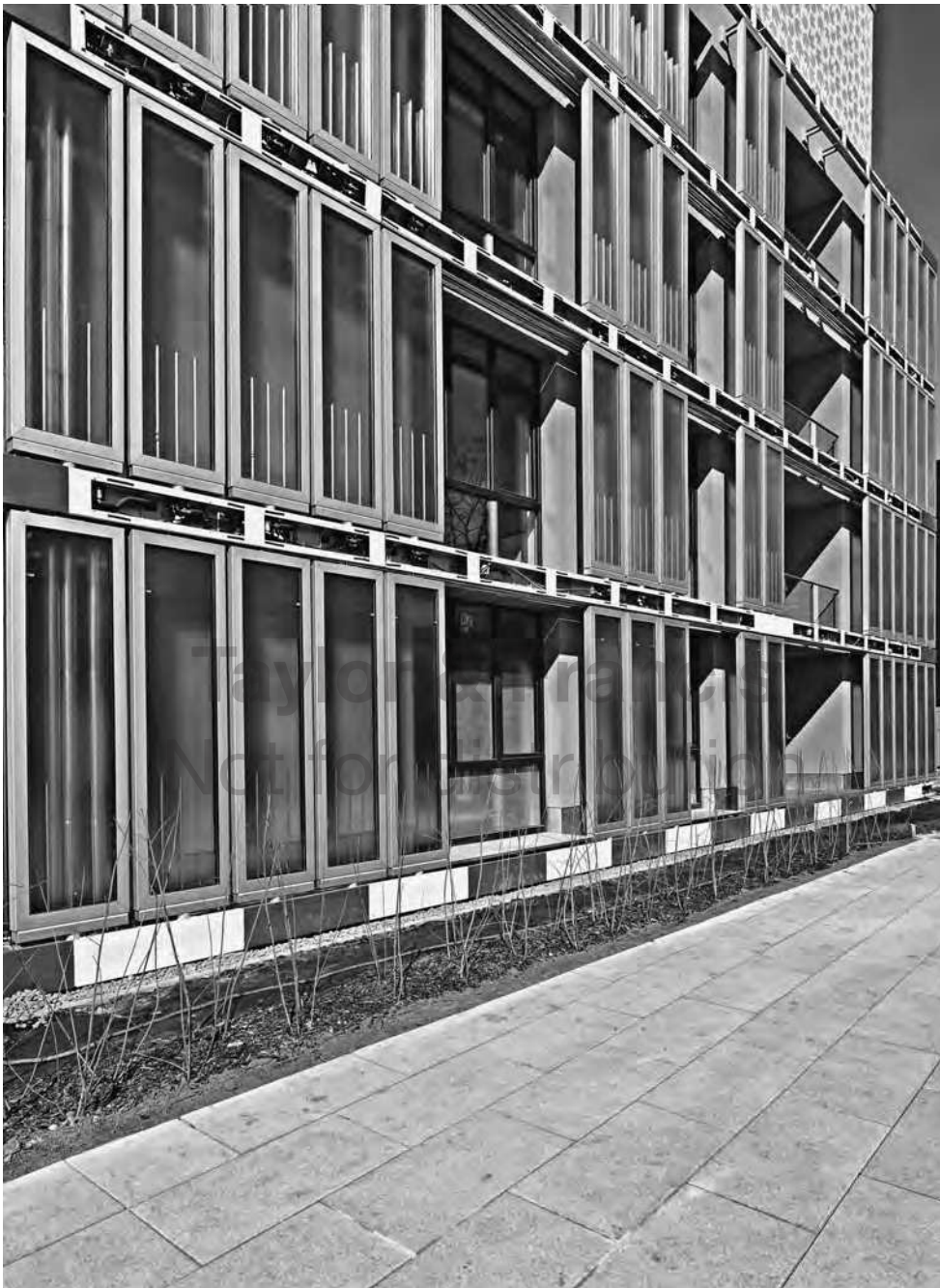
Figure 9.4 BIQ building, Hamburg, by Arup, exploits algae in façade Source: Arup Deutschland GmbH, Colt International GmbH and SSC GmbH)
