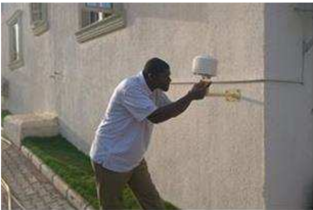
Fig 5: Installation of Tiny Tag external data loggers
