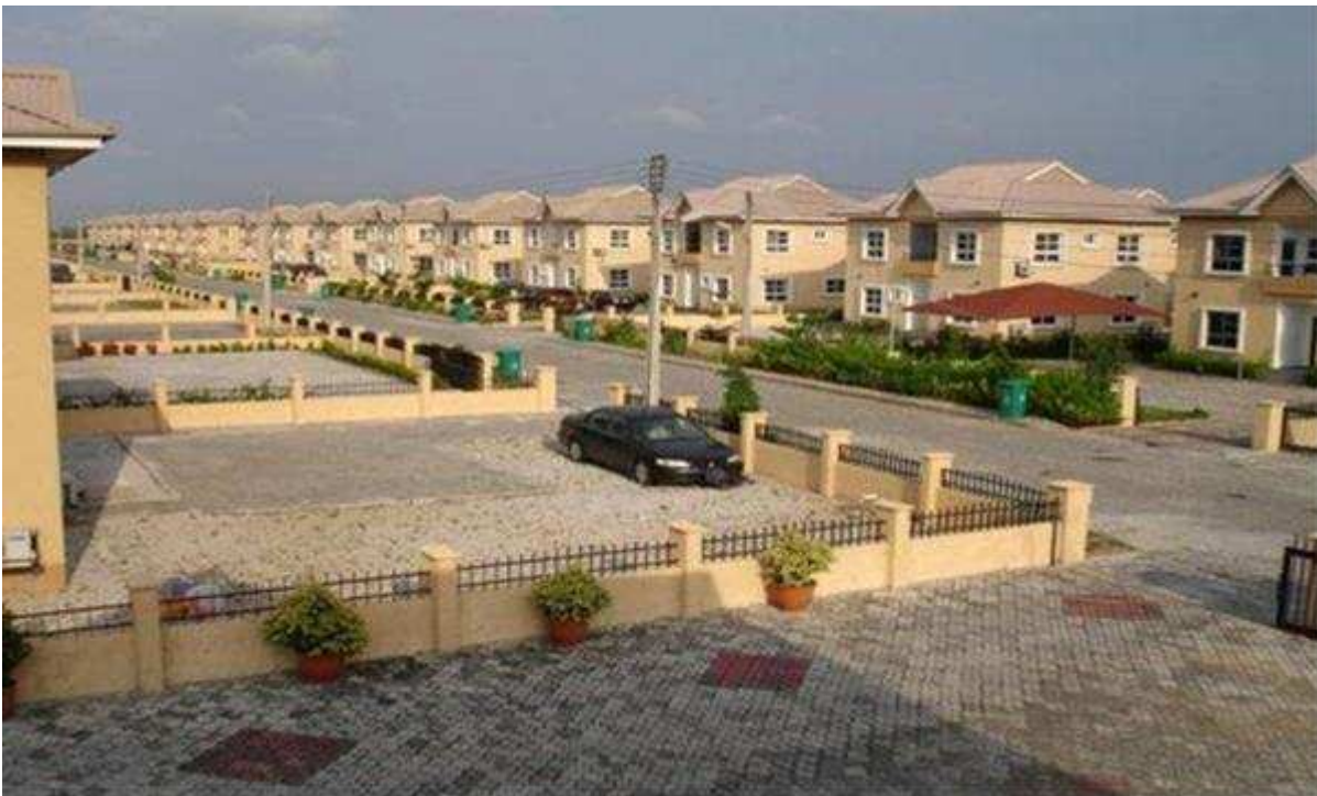
Fig 3: A typical medium-high income residential area in Abuja, Nigeria
