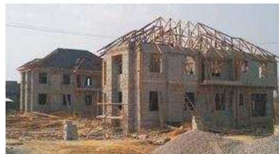
Fig 2: Building construction in Nigeria
