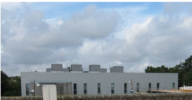
Fig 3: The ventilation stacks of the Jarman building
