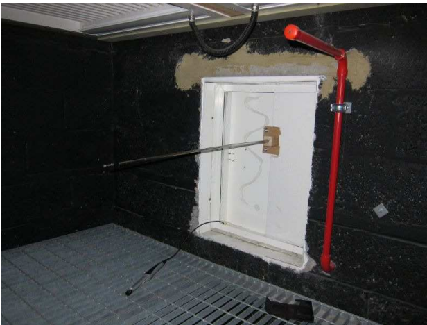
Fig 6: The top of the stack where air velocity, temperature and carbon dioxide were measured.
