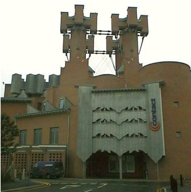
Fig 2: The naturally ventilated Contact Theatre, UK
