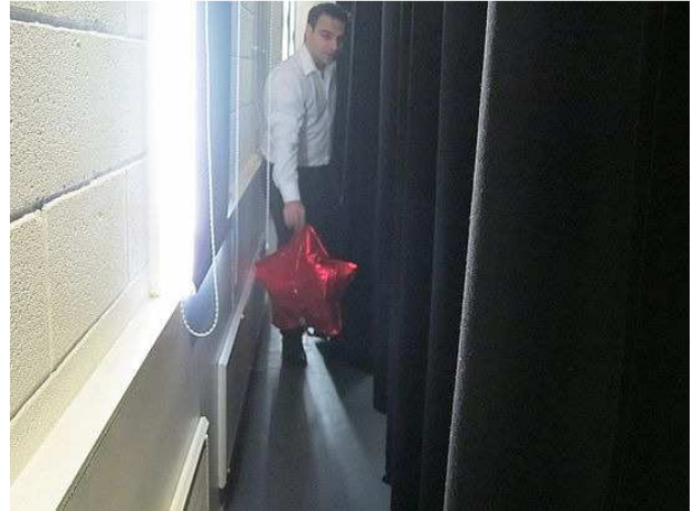
Fig 4: Testing behind the curtains, and showing the perimeter Passivent air inlet grilles
