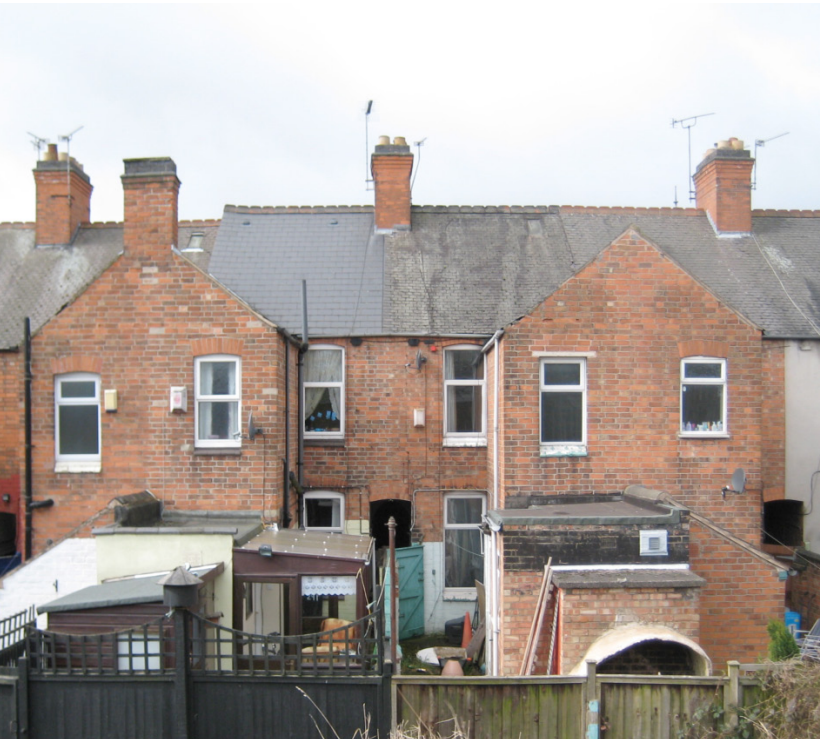
Figure 3: Terraced housing, which is superficially easy to renovate and insulate is, in the detail, surprisingly complex, especially at the rear.
