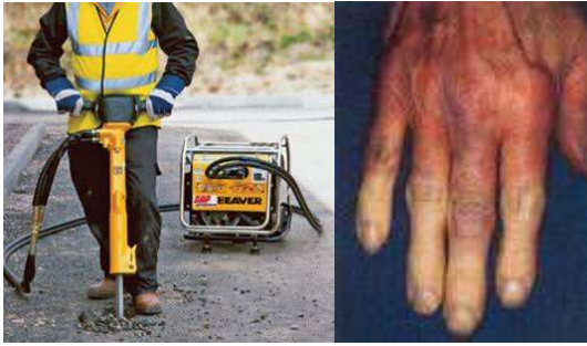
Figure 1: Left: A pneumatic drill in operation. Right: An operative's hand with white knuckle syndrome as a result of extended exposure to hand-arm vibrations.
