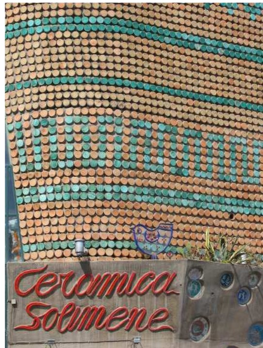
5.2.3. Detail of the façade (current condition)
