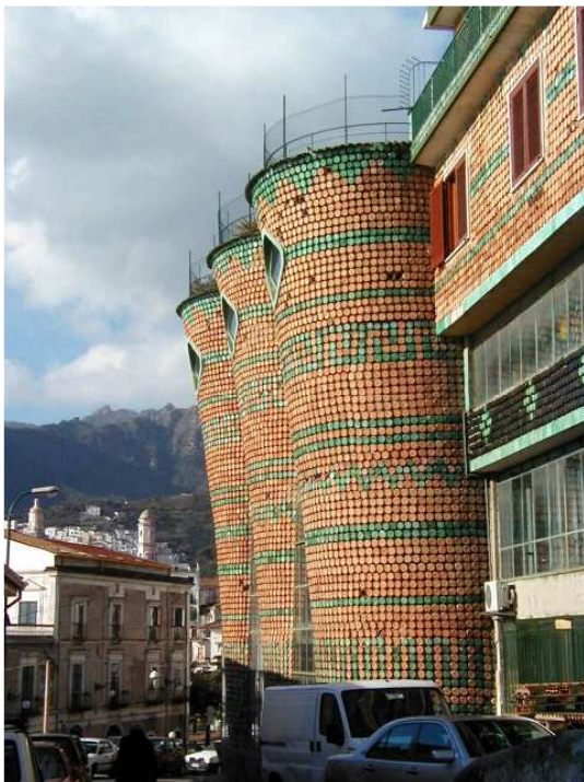
5.2.2. External view (current condition)
