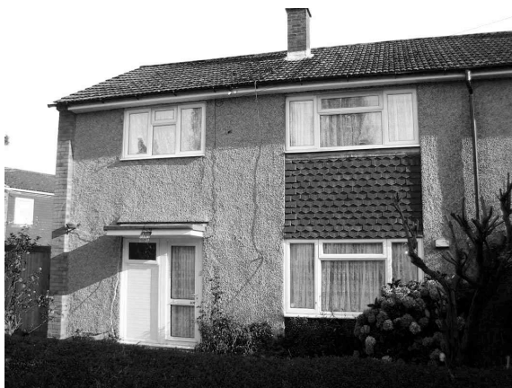
Figure 2: The Nine Acres house, constructed in 1950's using the Wimpey no-fines method
