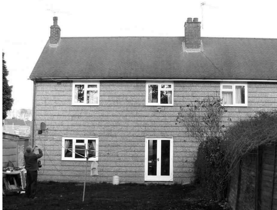
Figure 1: The Chester house – constructed in 1947 using the Airey method, comprising concrete studs and pre-cast concrete ‘weatherboarding’
