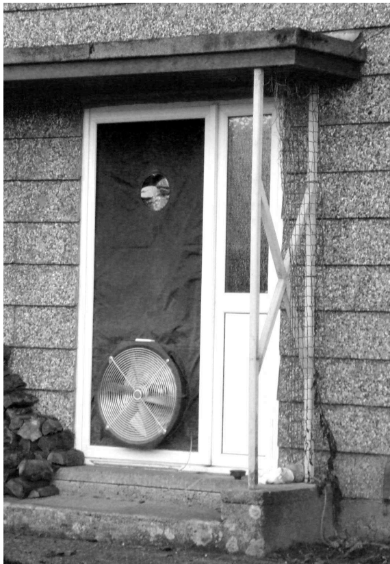
Figure 4: Air pressure testing was carried out at all three properties
