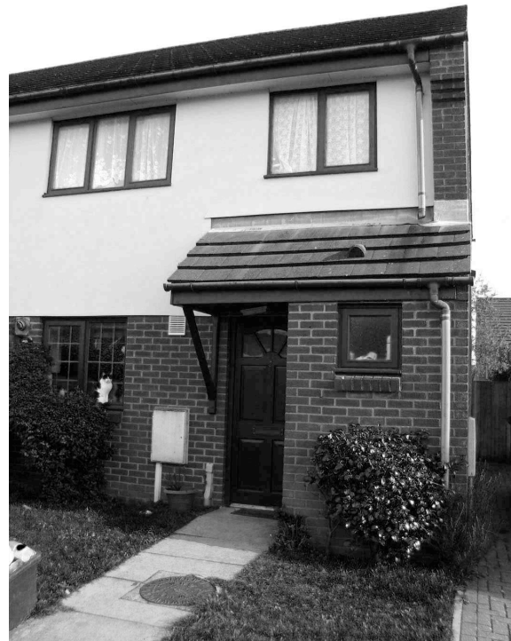
Figure 3: Photograph of Grebe – with render and brick-faced cavity wall construction typical of many thousands in the UK
