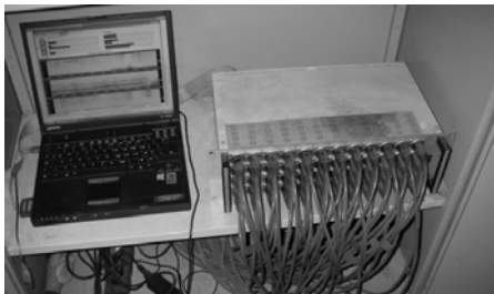
Fig.2 Flame stability monitoring system in operation
