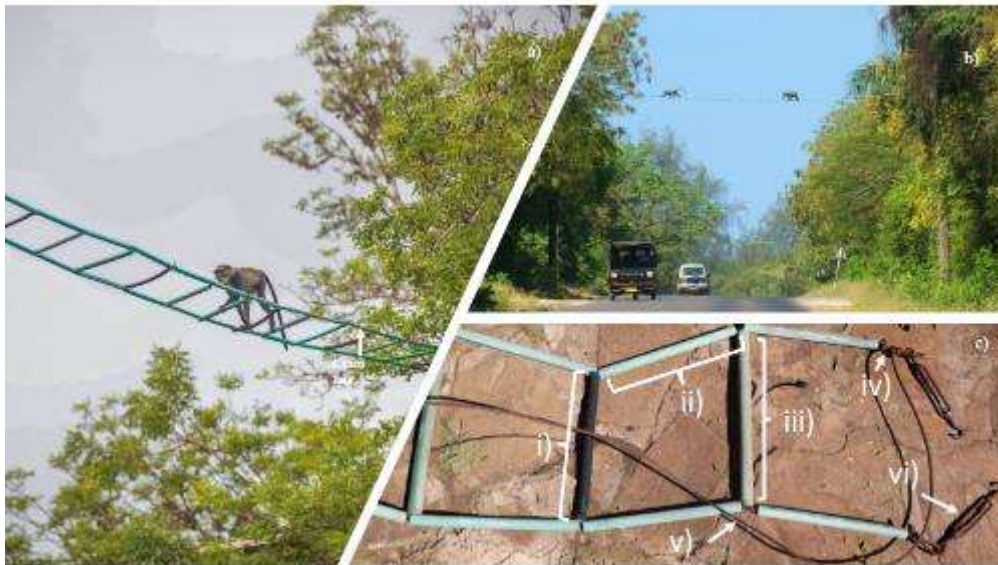
Figure 3.1 Horizontal ladder canopy bridges over Diani's Beach Road. a) Sykes' monkey crossing with bridge rungs visible, b) two Sykes' monkeys crossing, c) bridge components are: i) 30 cm rubber pipe, ii) 30 cm PVC conduit pipe, iii) 45 cm pressure pipe, iv) 3/16" galvanized wire rope grips, v) 3/16" galvanized wire, vi) turnbuckle. Photos a) and b) by 2 nd author Andrea Donaldson, photo c) Colobus Conservation photo library.
