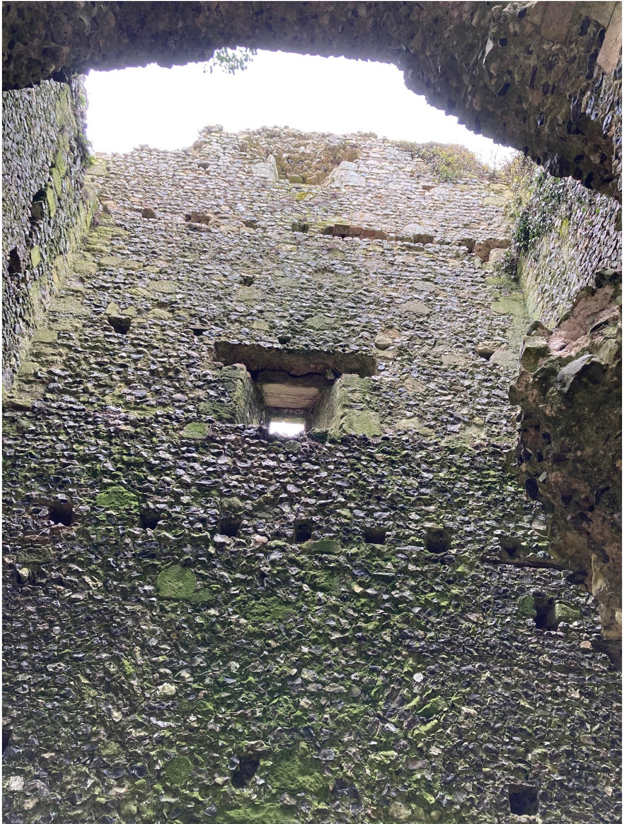
Interior view of the remaining tower
