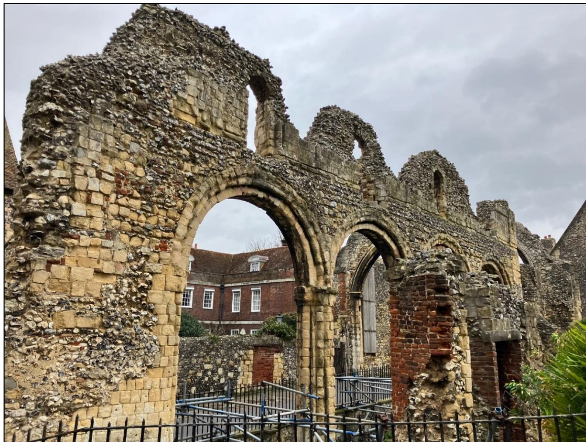
Fig. 21 Fig: A heavily consolidated section of damaged walling from Christ Church Priory Infirmary remains standing on the grounds behind the Cathedral, (photo author, 2022).
