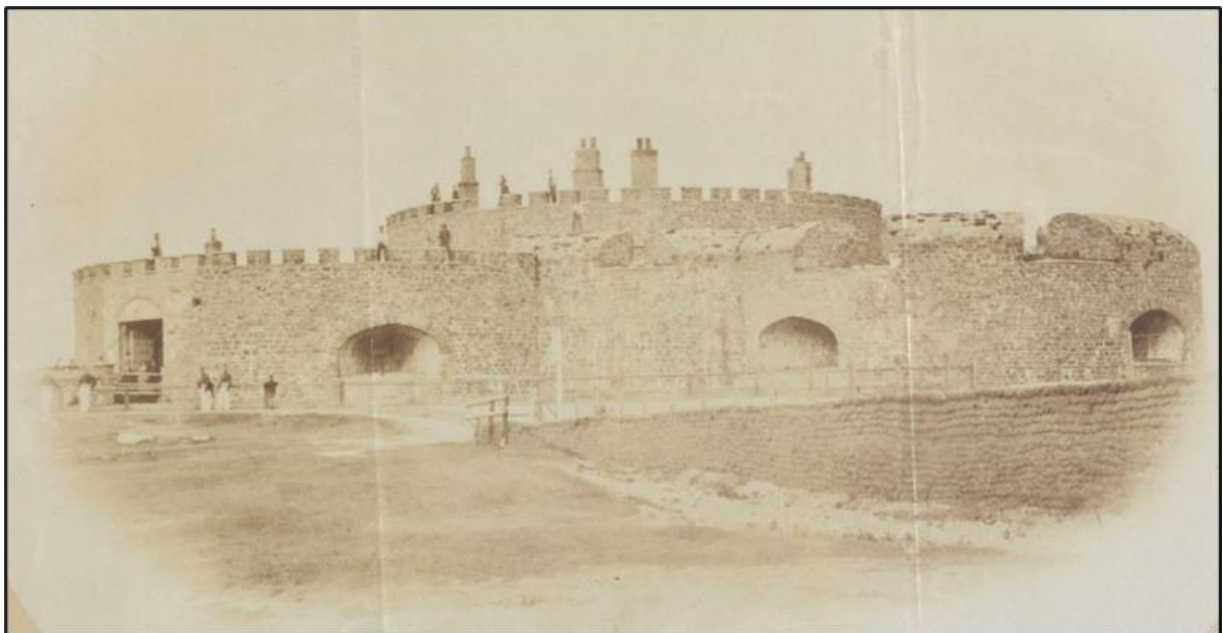
Fig. 14 Photo showing the newly constructed sea wall butting up to the old fortress (the view is from the West, therefore the beachside is to the right of this photo), 1863, The National Archives, WORK36/124.
