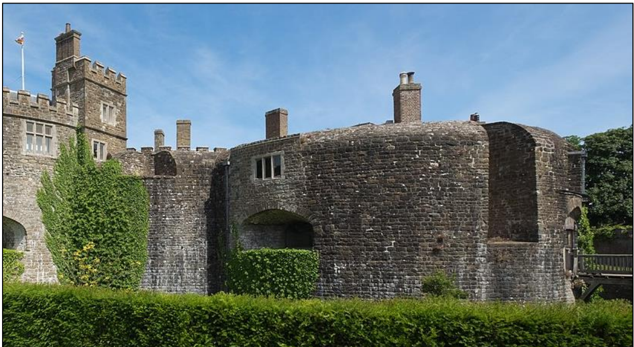
Fig. 10 Photograph of the landward (westerly) bastion at Walmer Castle showing the deep splayed embrasures, (photo author, 2019).
