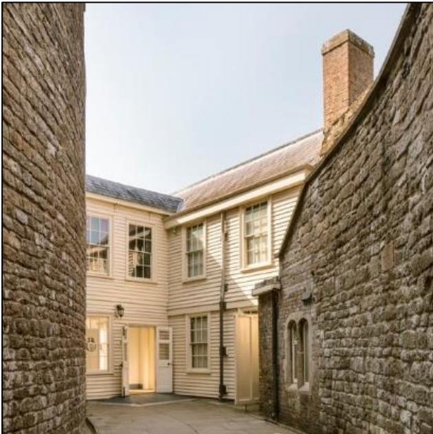
Fig. 6 Gunners' Cabins, Photograph taken following the 2015 refurbishment, 2016, Historic England Archives, DP261562.
