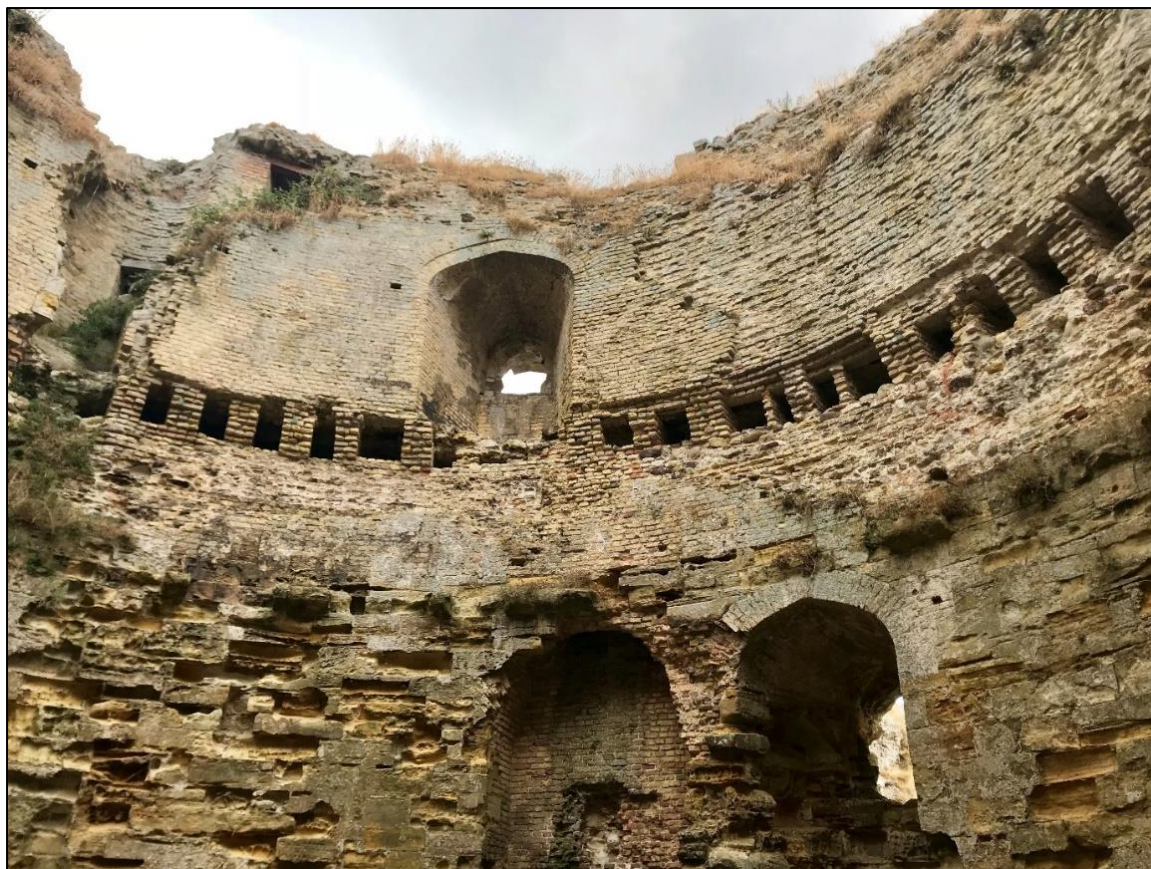
Fig. 26 The interior of the keep at Camber Castle, (photo author, 2018).
