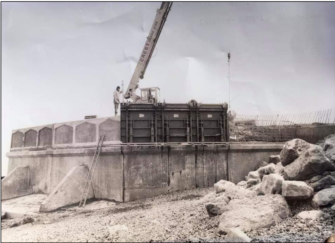
Fig. 33 Sea defences being installed into the ruins of Sandown Castle, c. 1980s, used with permission of Mrs Linda Ford Chair of Sandown Castle Community Garden, Private Collection (Unpublished).
