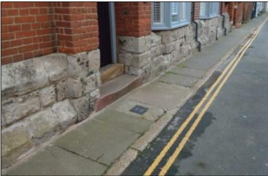
Fig. 60 Side elevation of the reading rooms building in Deal showing how the Sandown stones have been incorporated to build a plinth on the building, 2019, © Google Street View, used under UK fair dealing.
