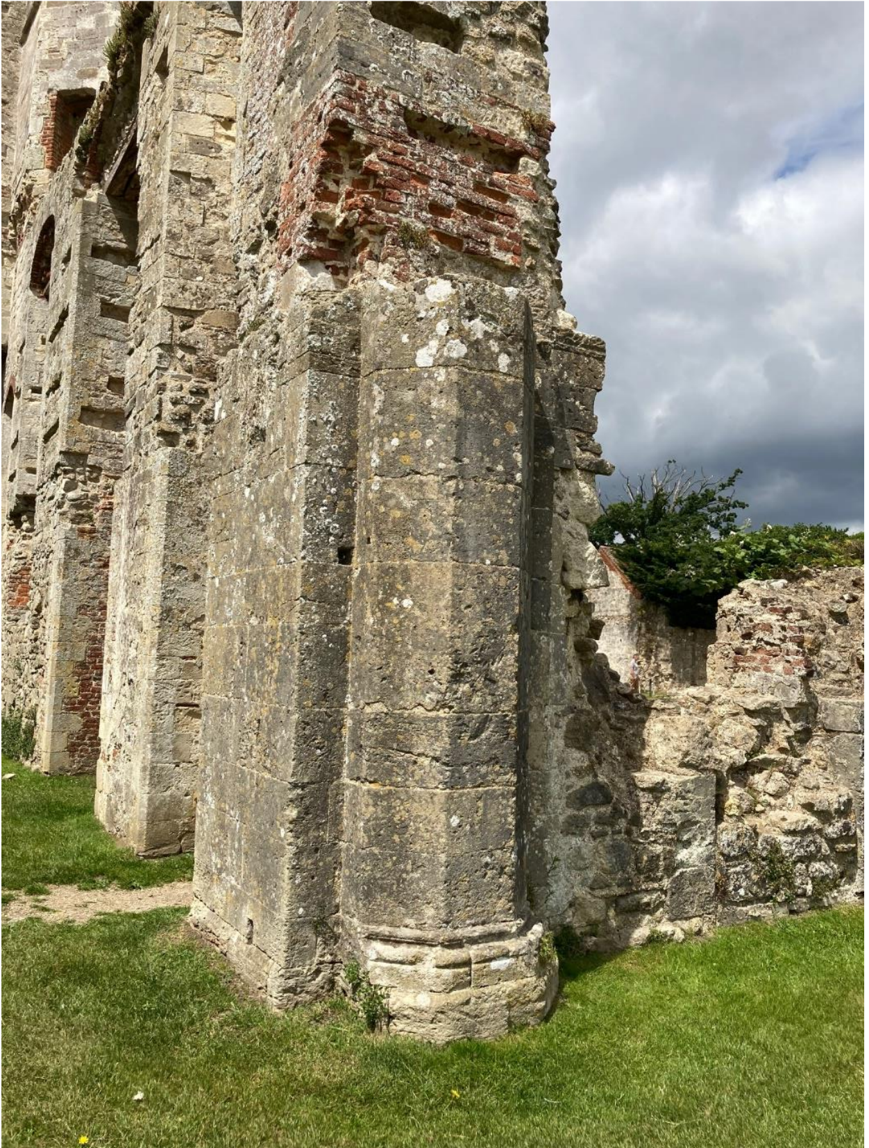
Remains of a column affixed to the front elevation
