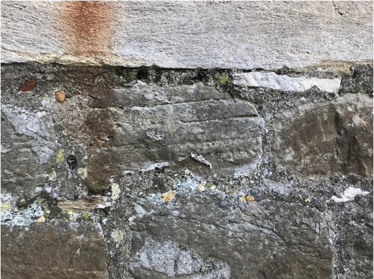
Apparent signs of a variety of differing spolia with former mason tool markings
