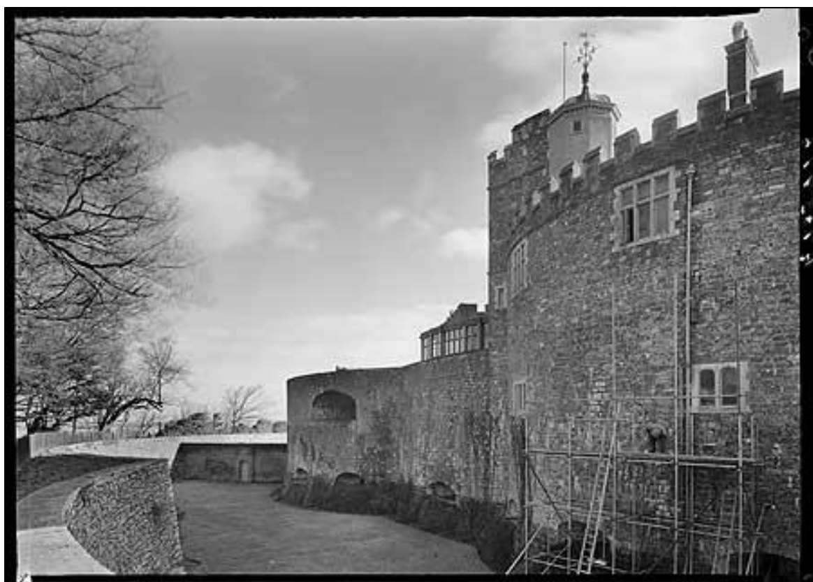
Fig. 75 Scaffolding being erected for repointing works, 1966, Historic England Archives, P/A07039/006.
