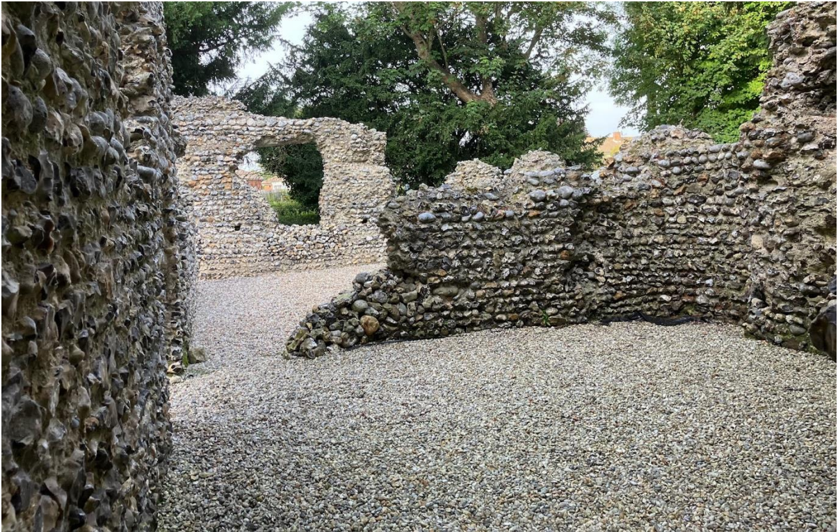
The interior of where the keep would have been built
