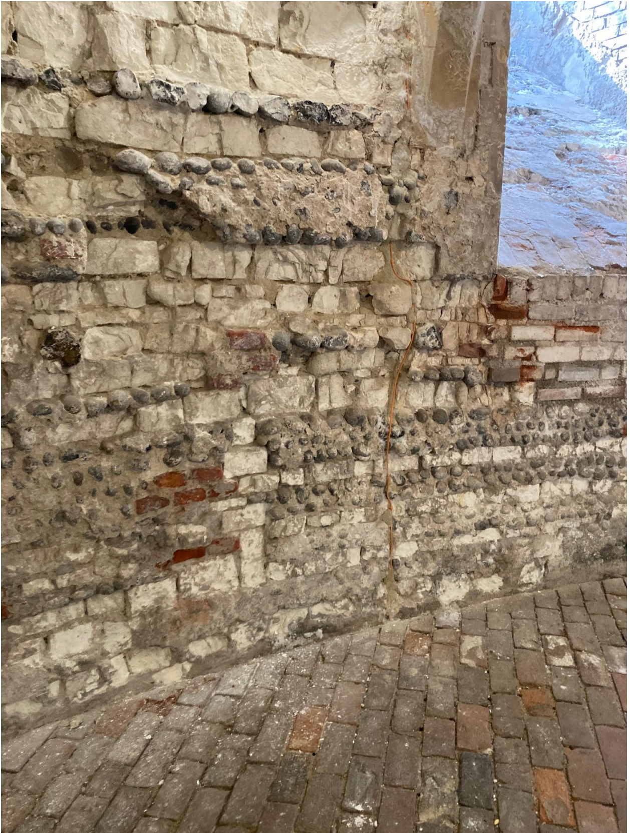
Spolia, flint, and CBM used in the keep's basement walling
