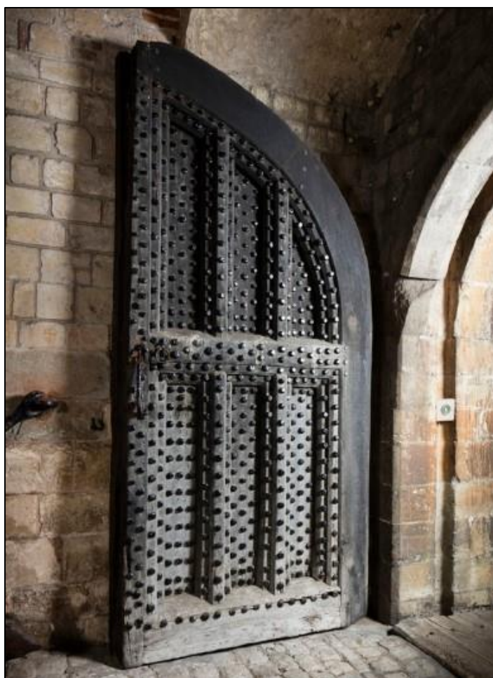
Fig. 46 Detail of the Castle's studded door in the main entrance passage, Historic England, 2016, DP187736.
