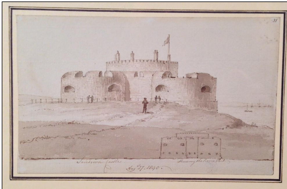
Fig. 7 A sketch by Henry Moses in 1840 depicting Sandown Castle, held in a private collection.
