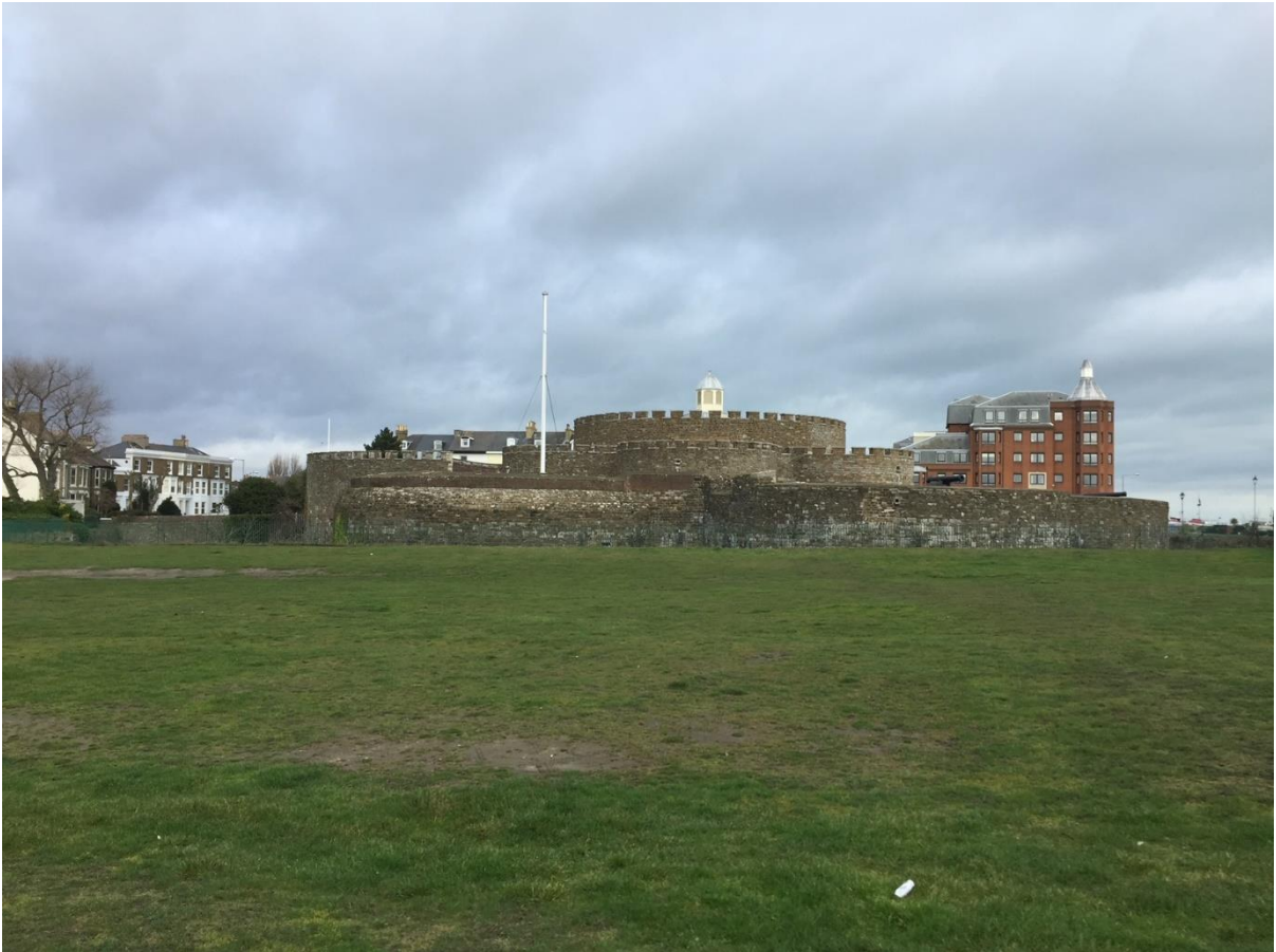
View north from the carpark
