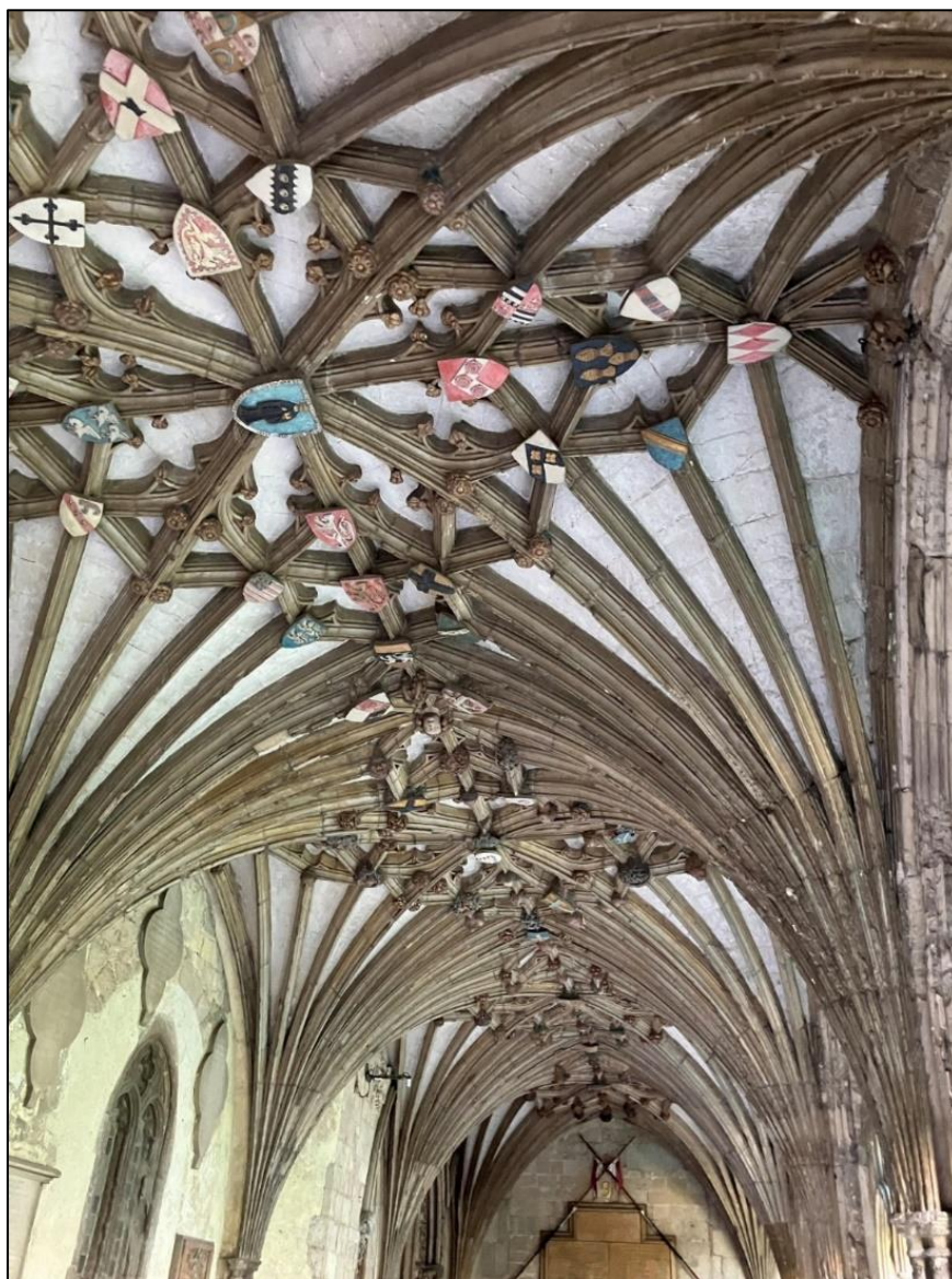
Fig. 66 The remaining cloisters at Canterbury Cathedral, showing the vaulted ribwork that is said to be Purbeck Marble (photo author 2023).
