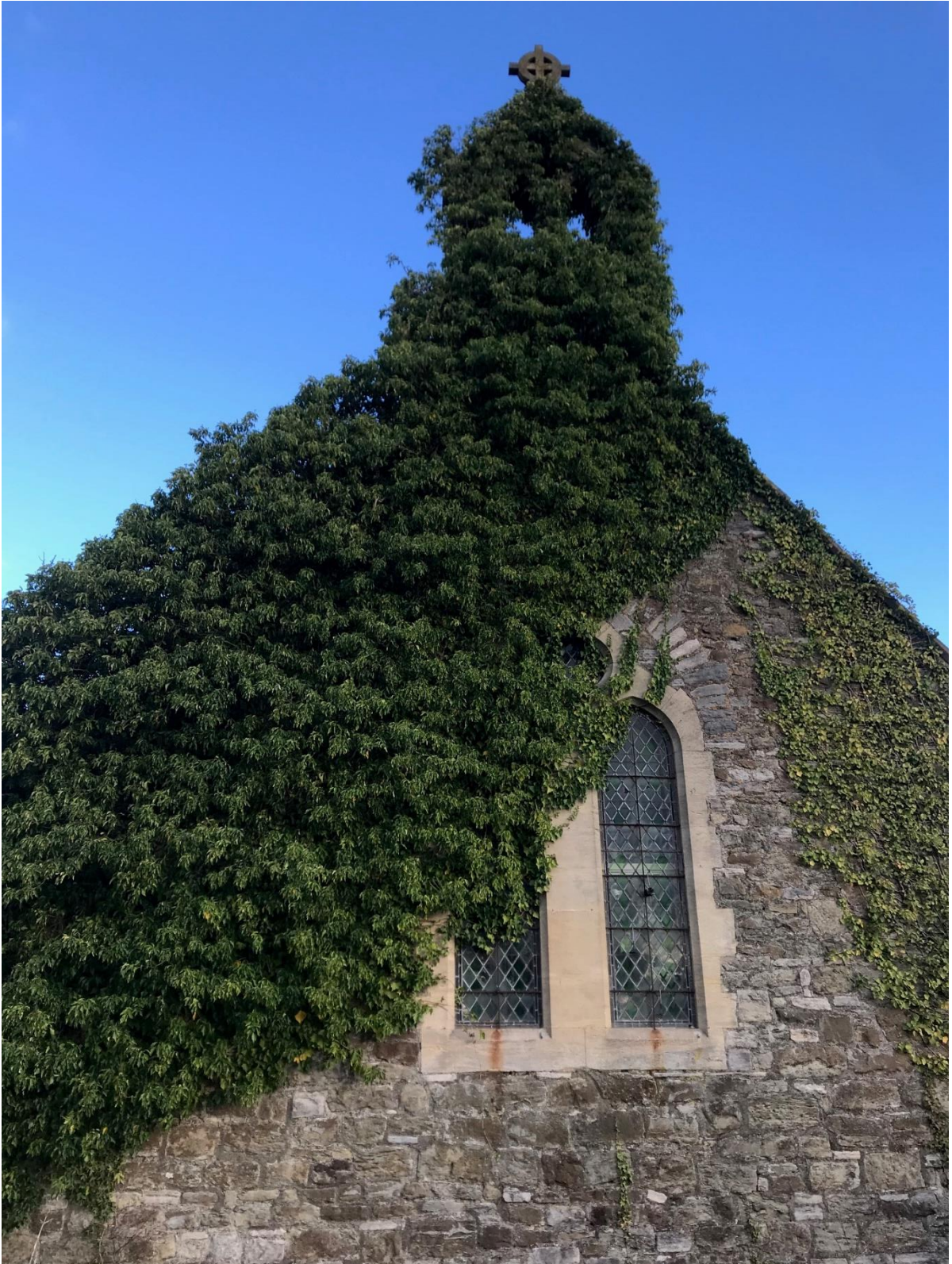
Vegetation taking hold on the southern flank
