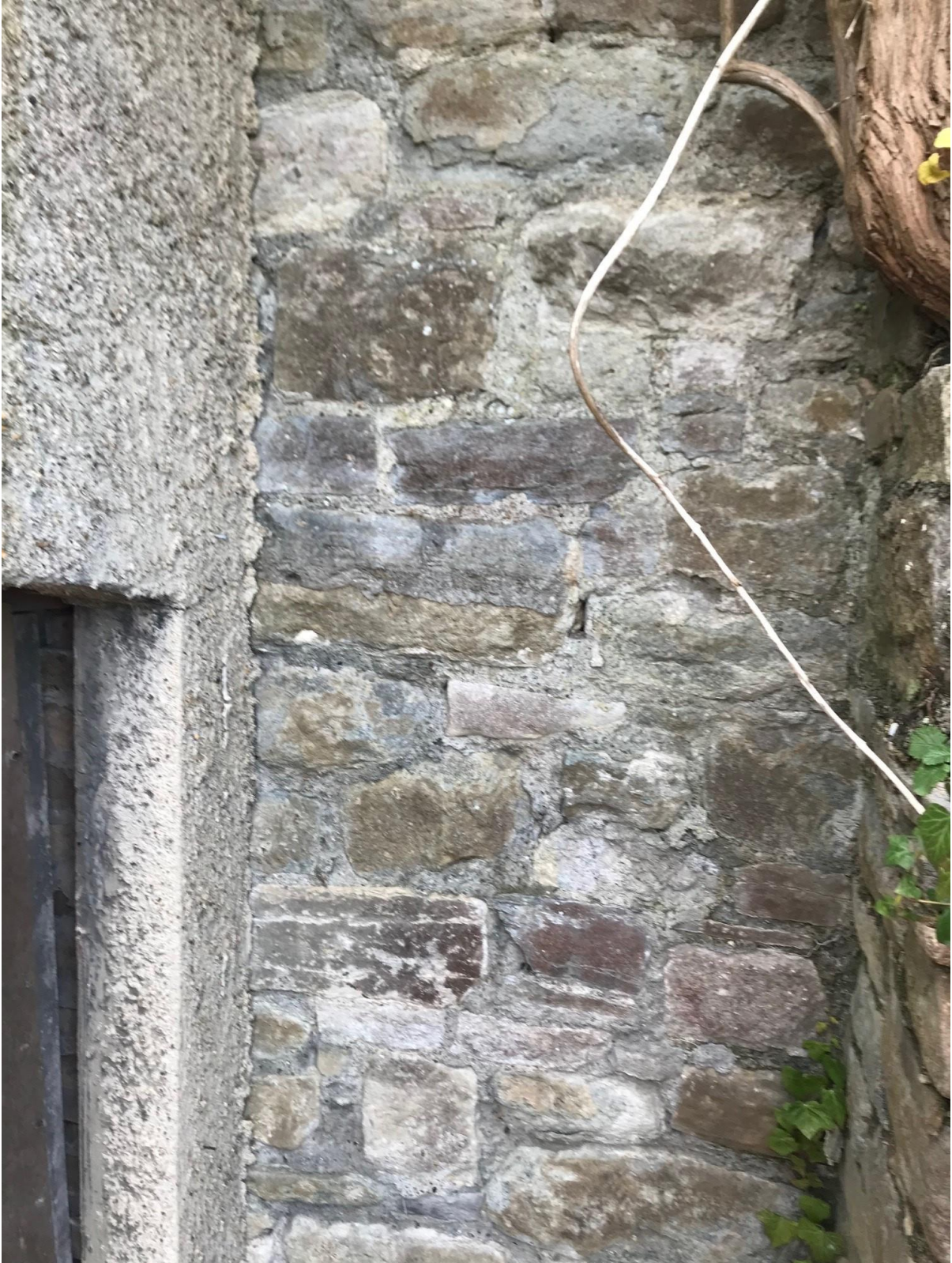
Example of Kentish Ragstone (et al.) within the walling, all probable spolia examples.
