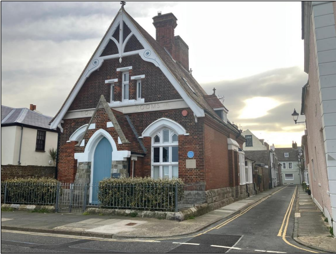
Fig. 59 Boatmen's Rooms, 182 Beach Street, Deal Kent (photo author, 2024).
