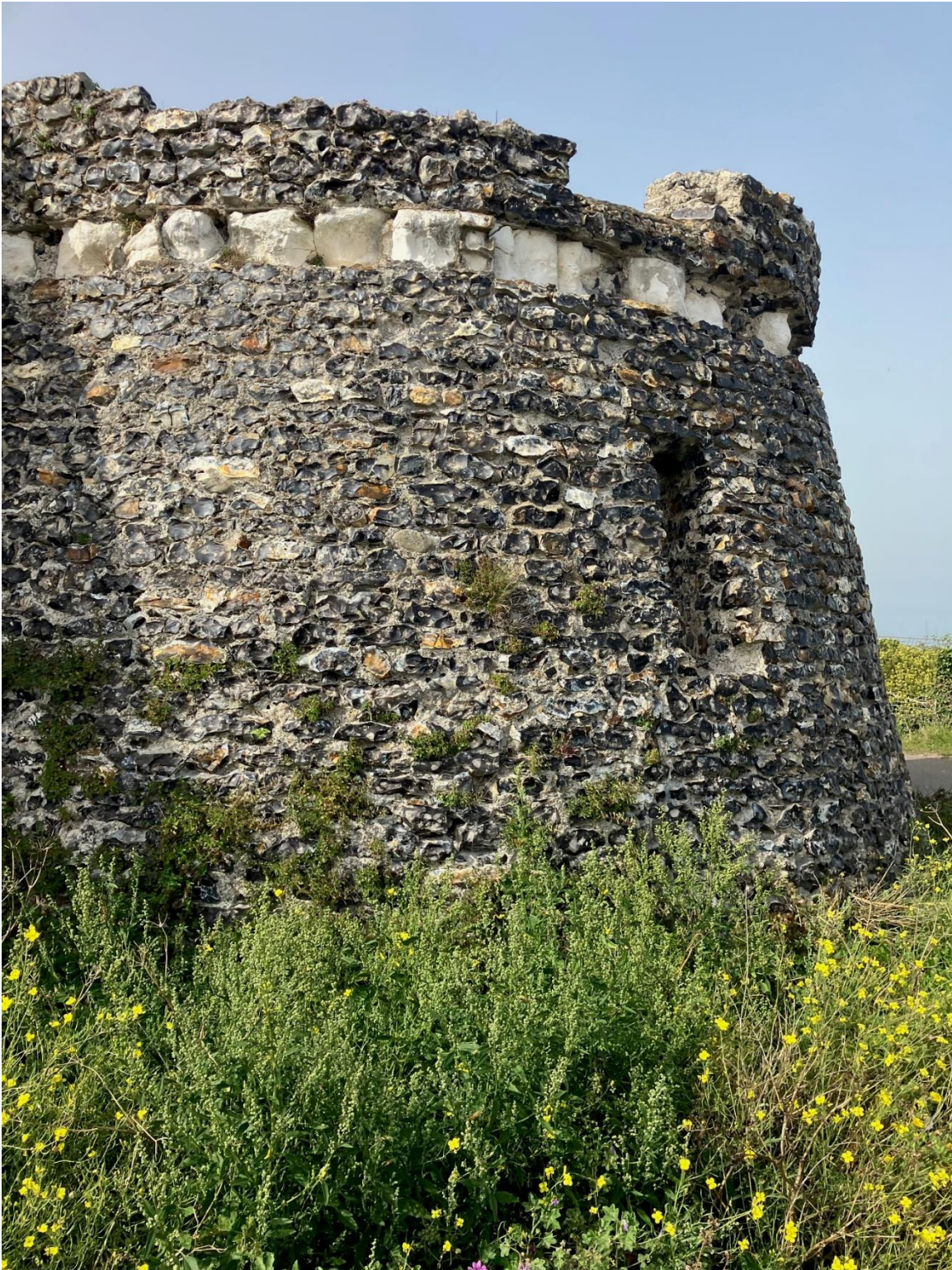
Chalk coursing to this 'bastion' with flintwork walling
