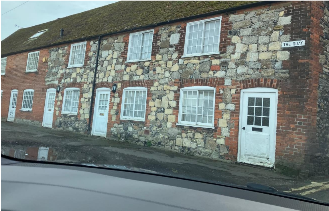
Various reused stones in the elevation of these cottages
