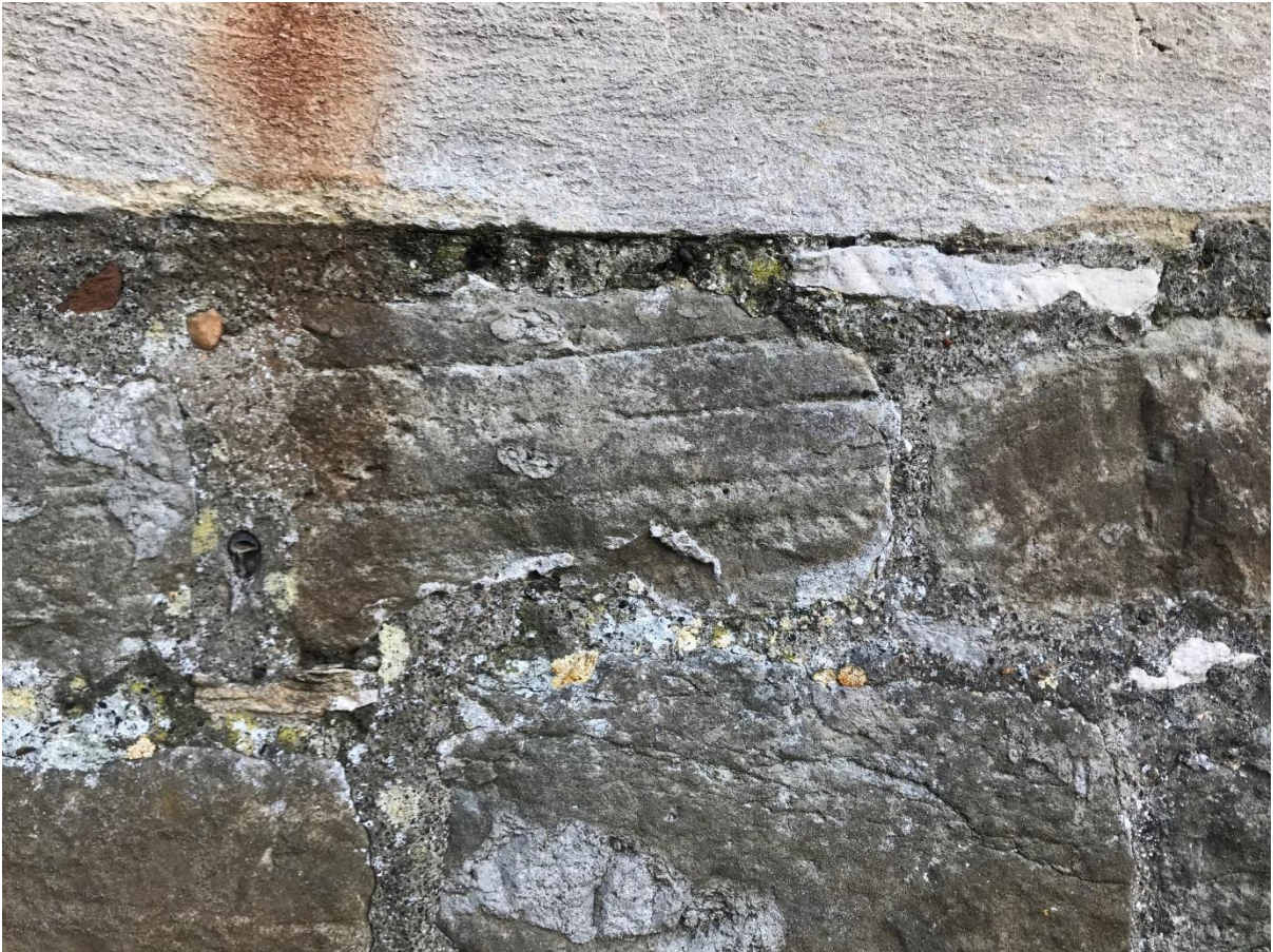
Example of spolia/medieval masonry markings in the main chapel elevations as probably taken from St Radegunds Abbey via Sandown Castle
