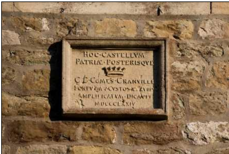
Fig. 42 Fig: A plaque installed at the end of the extensive Granville alterations, located above the entrance in the main entrance bastion, c. late twentieth century photograph, Historic England Archives, DP165356.
