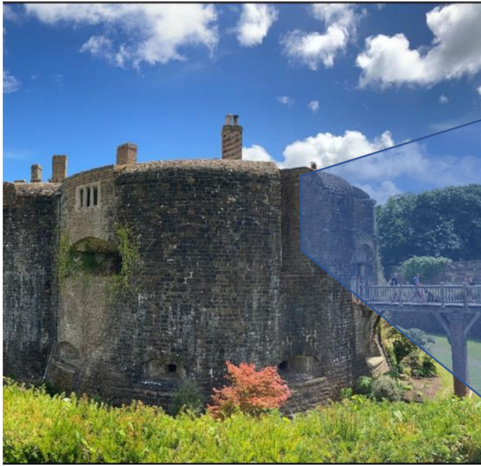
Fig. 41 Walmer Castle with one of its less-altered bastions, showcasing the reduced coverage due to the restrictive parapet embrasures, (photo author, 2022).
