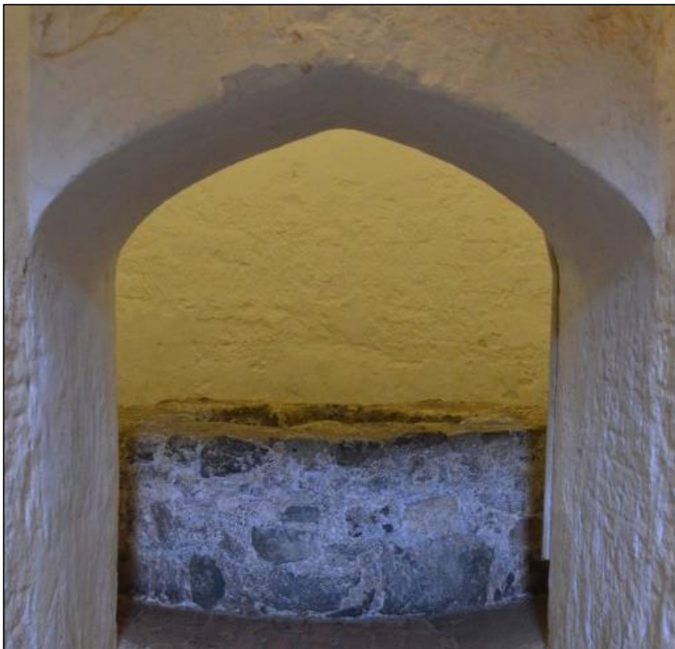
Fig. 9 The original Tudor well in Deal Castle's Keep, (photo author, 2018).
