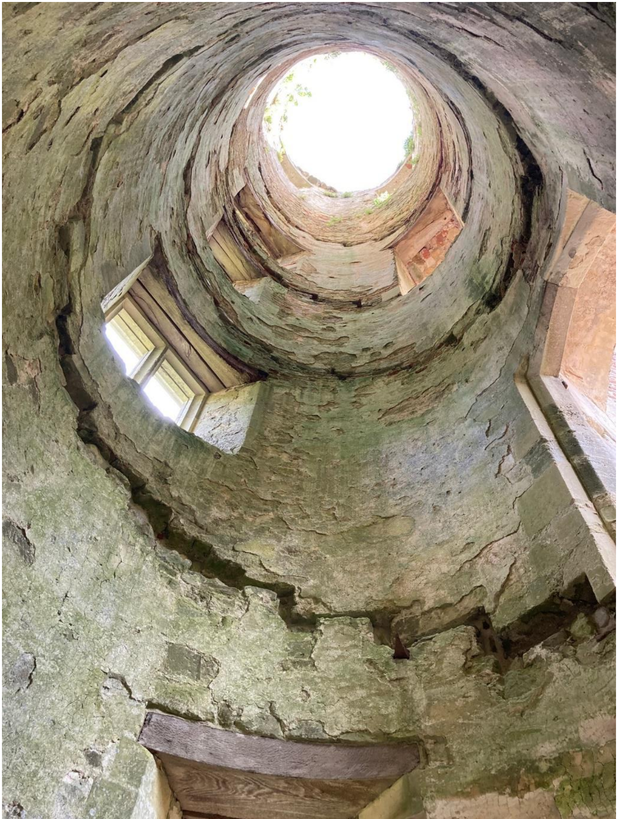
View of the interior of the tower
