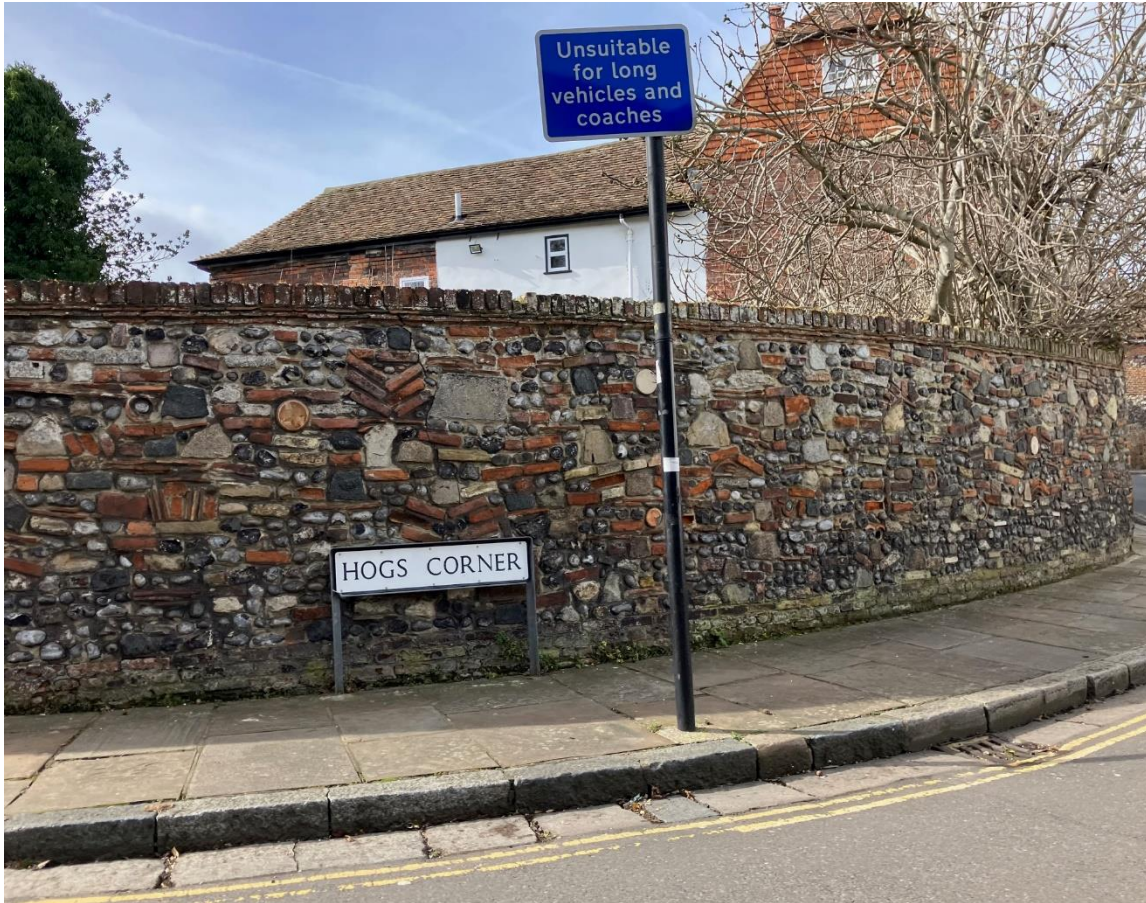
Example of spolia using stone and CBM to this garden walling to The Salvation
