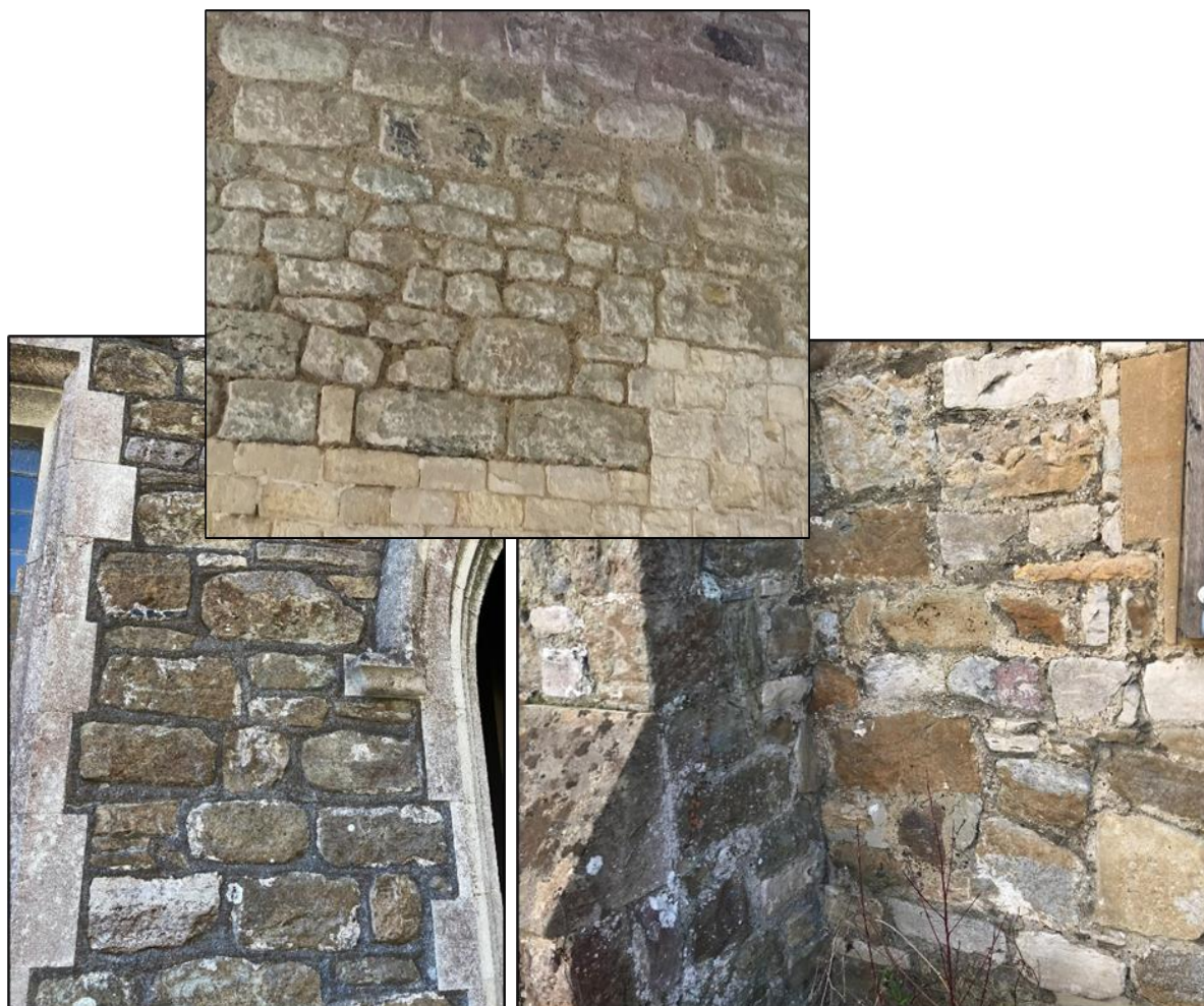
Fig. 65 Photographs taken by the author. Top left: Constable's Tower, top right: Eastry Chapel, below: Walmer Castle's entrance bastion. All examples show reused spolia from Sandown Castle.
