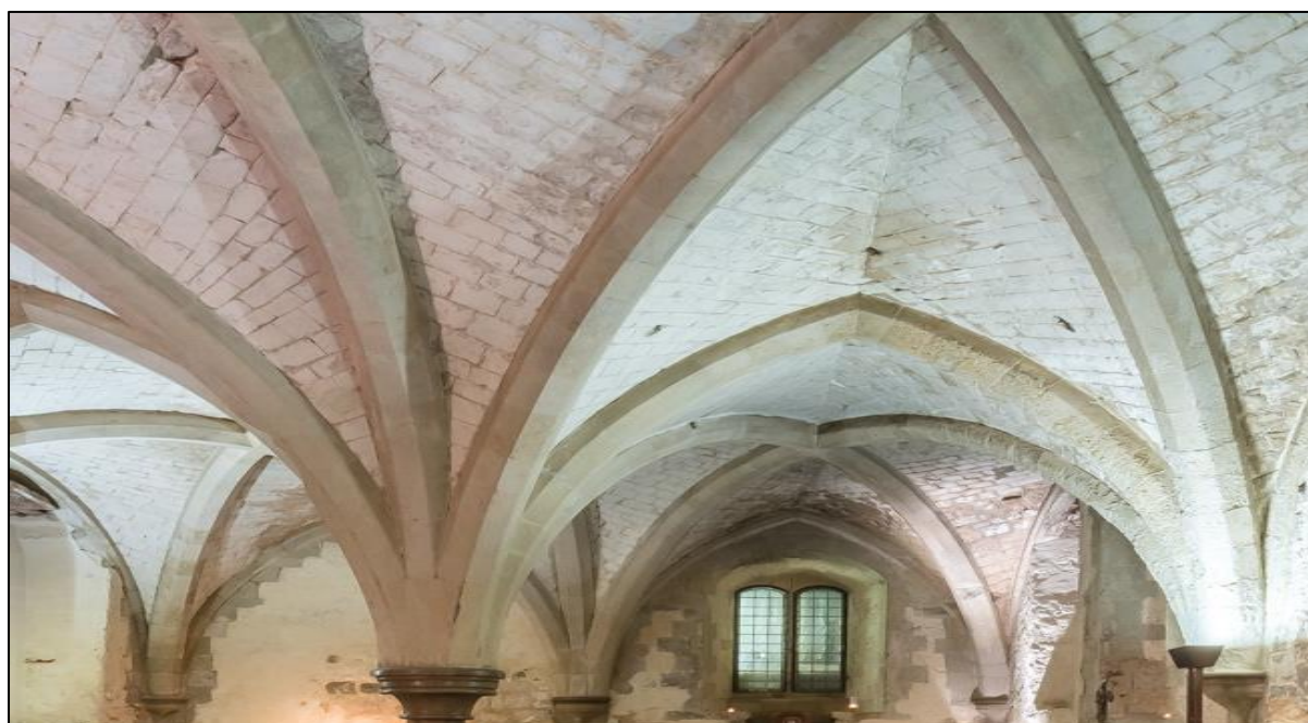
Fig. 13 The vaulted ceiling in Lambeth Palace's chapel, (photo author, 2018).
