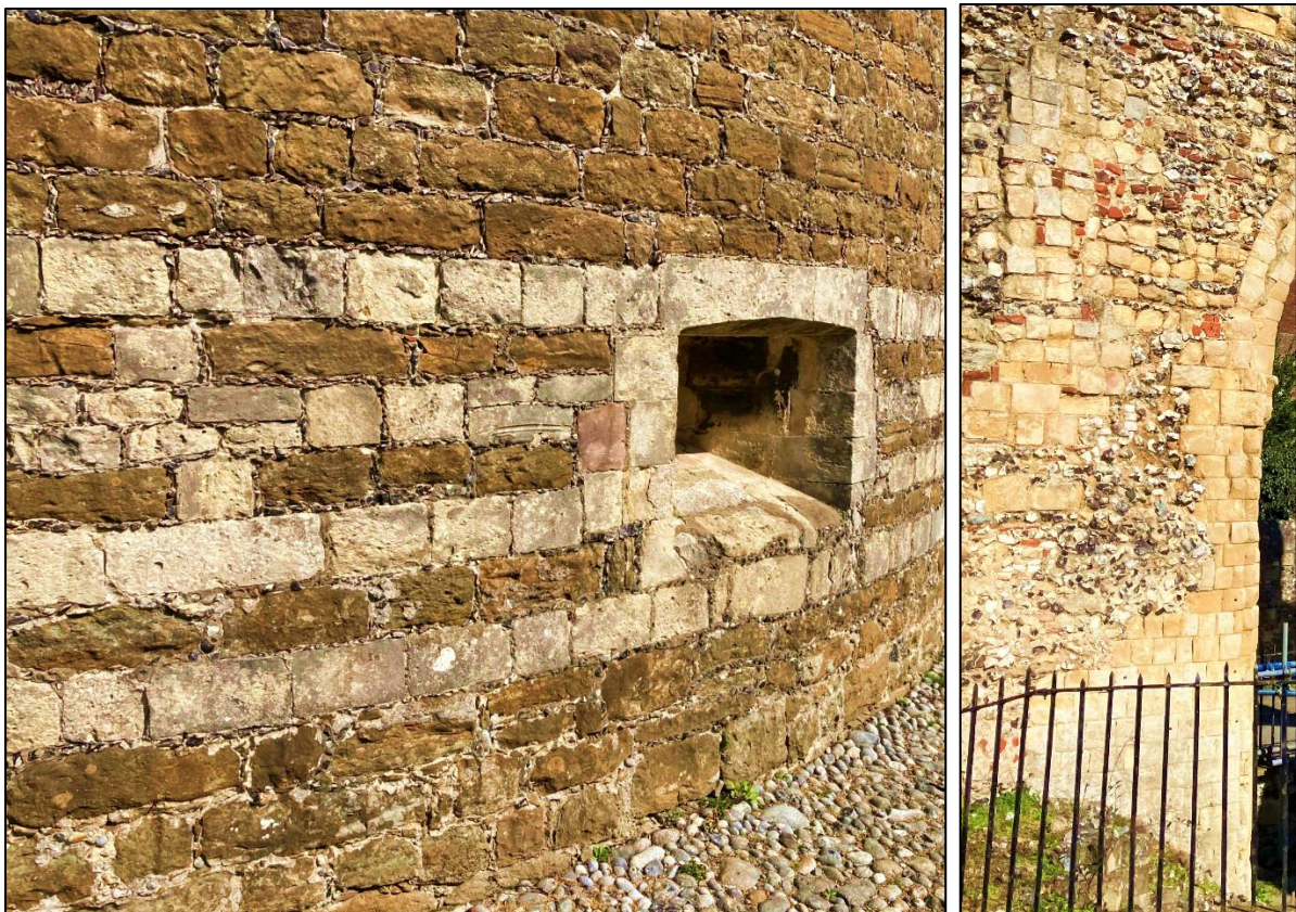
Fig. 5 Left: Photograph by the author of examples of spolia (possibly Caen) at Deal Castle, taken in 2020. Right: A photograph of Caenstone in situ at Canterbury Cathedral, as taken by the author in 2022.
