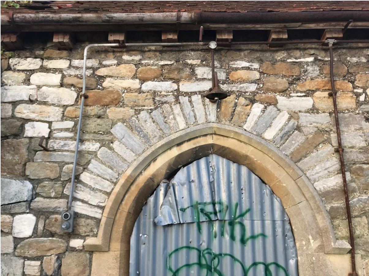
Example of spolia reuse stones to the curtain walling, arch stones possibly lifted from a doorway or ribbed ceiling at Sandown Castle. Note the vandalism.
