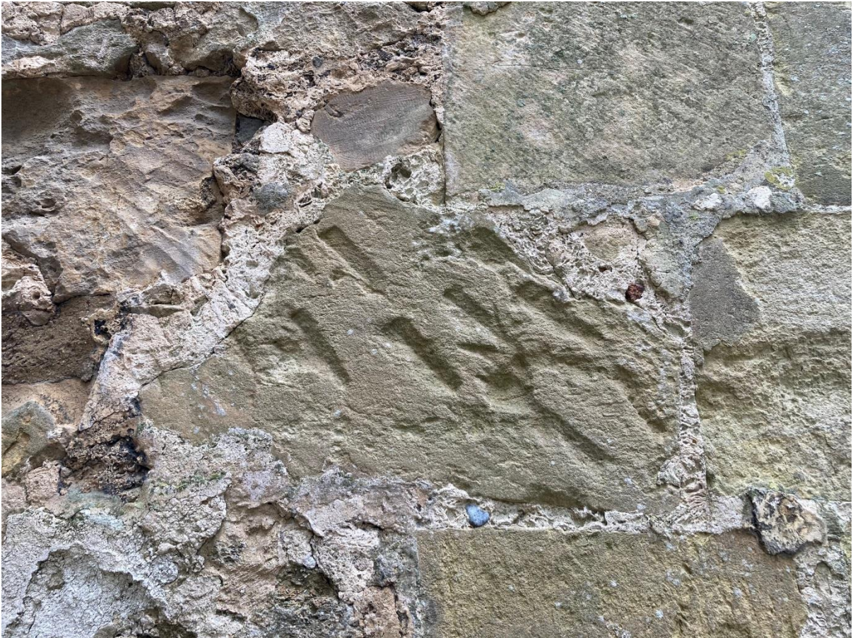
Mason's markings to the stonework used as a key for interior plasterwork since lost to time
