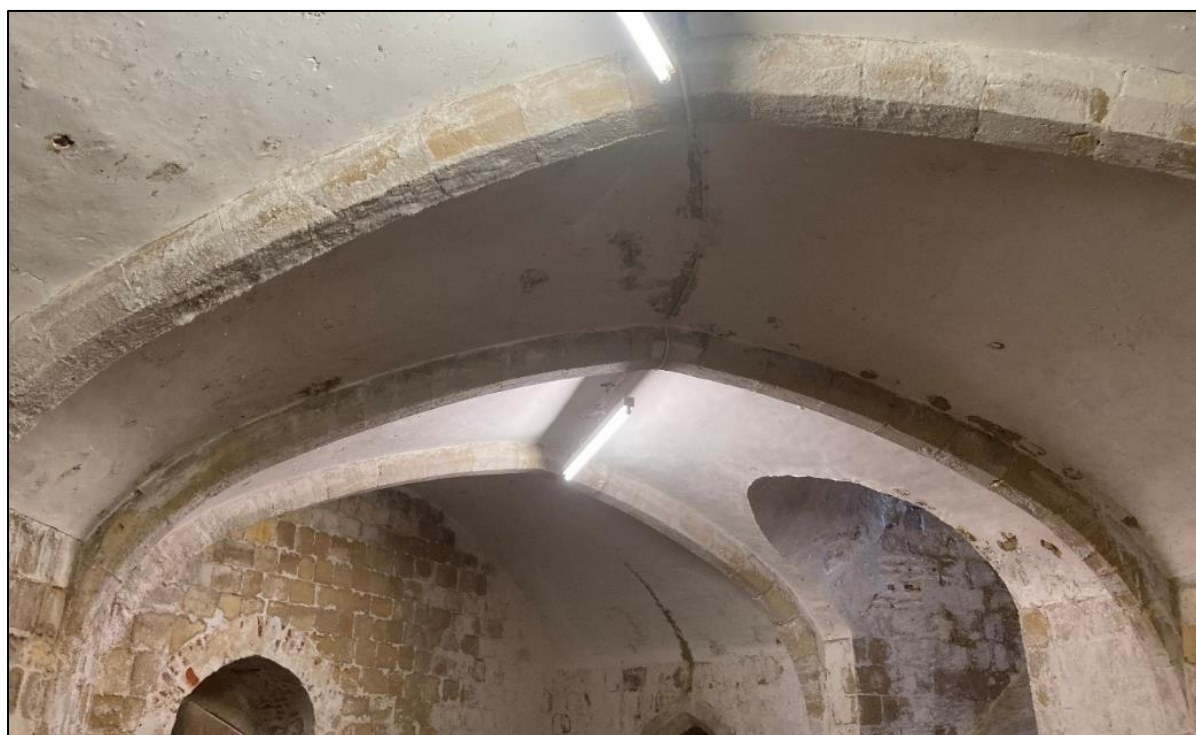
Fig. 12 The rib vaulting to Walmer Castle's keep basement, (photo author, 2018).
