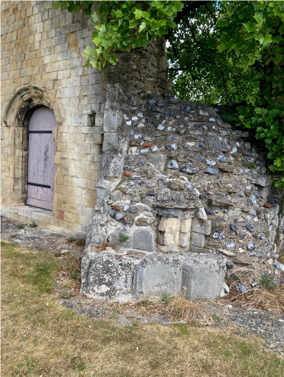
Consolidation work near the remains of the cloisters
