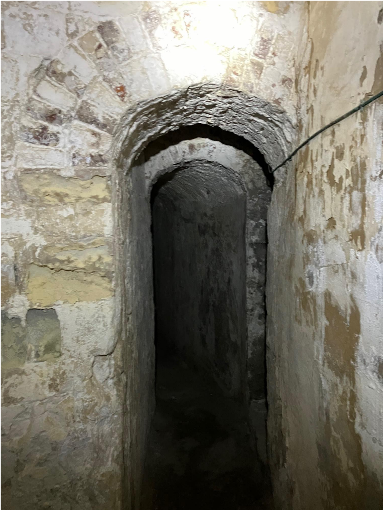
An example of the passageways that are nearly identical to the photographs from the 1980s of the Sandown Rounds. The passageways also demonstrate a significant quantity of original freestones (probably spolia) and Tudor bricks.
