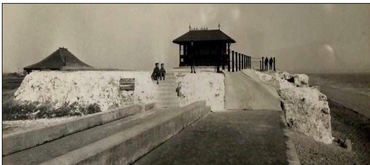
Fig. 30 Photograph showing the 'New walkway' at Sandown Castle with sea shelter, c. '1924', Deal Town Council Archive, CS765.
