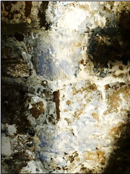
Fig. 17 Visible traces of 'Walmer Blue' coloured paint as found in 'The Rounds' of Deal Castle by the author in 2022.
