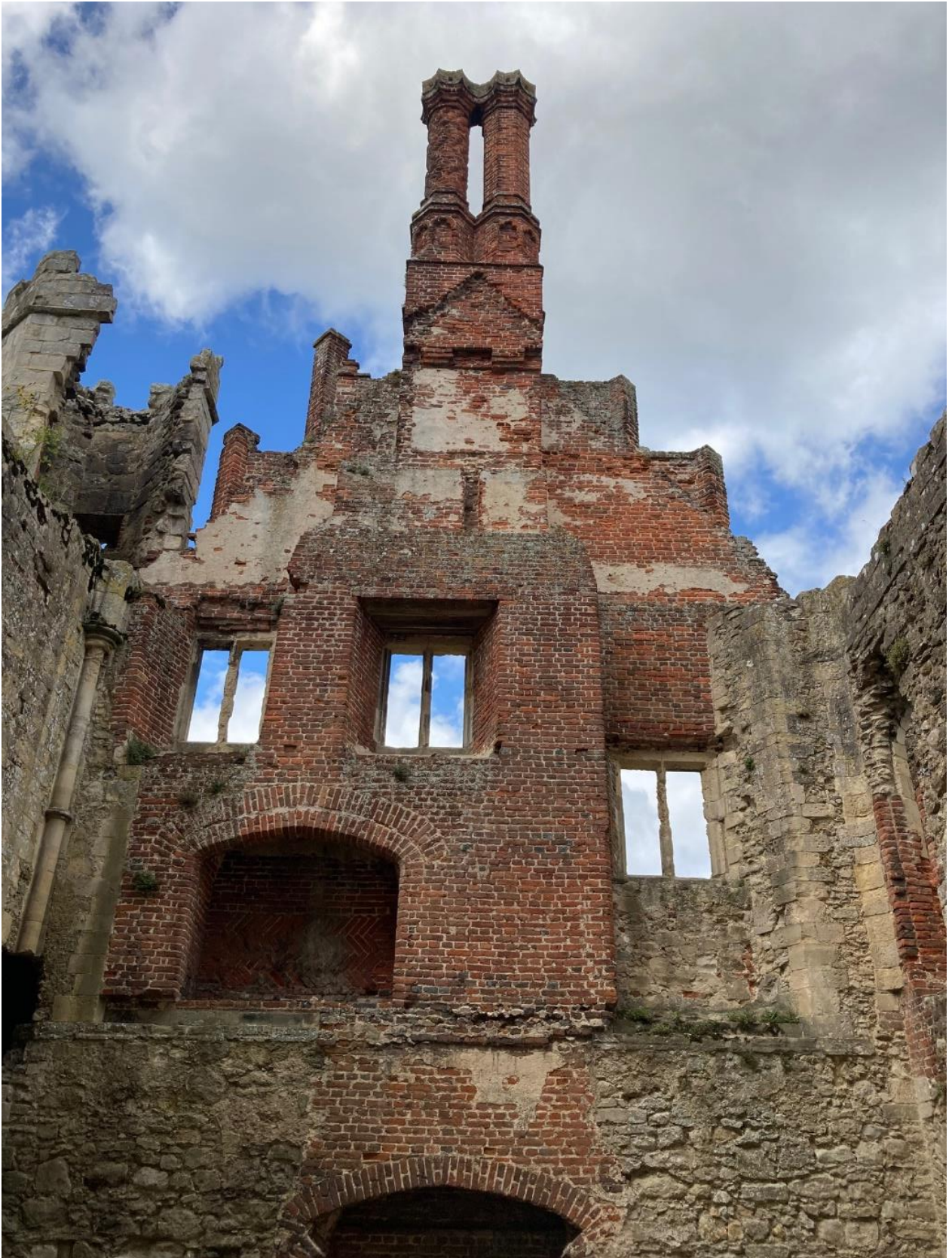
View of the interior face of the front elevation
