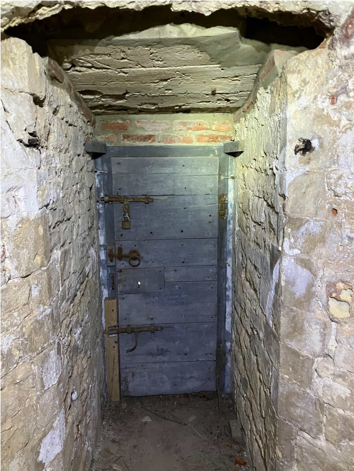
A modern exit formed below the drawbridge area
