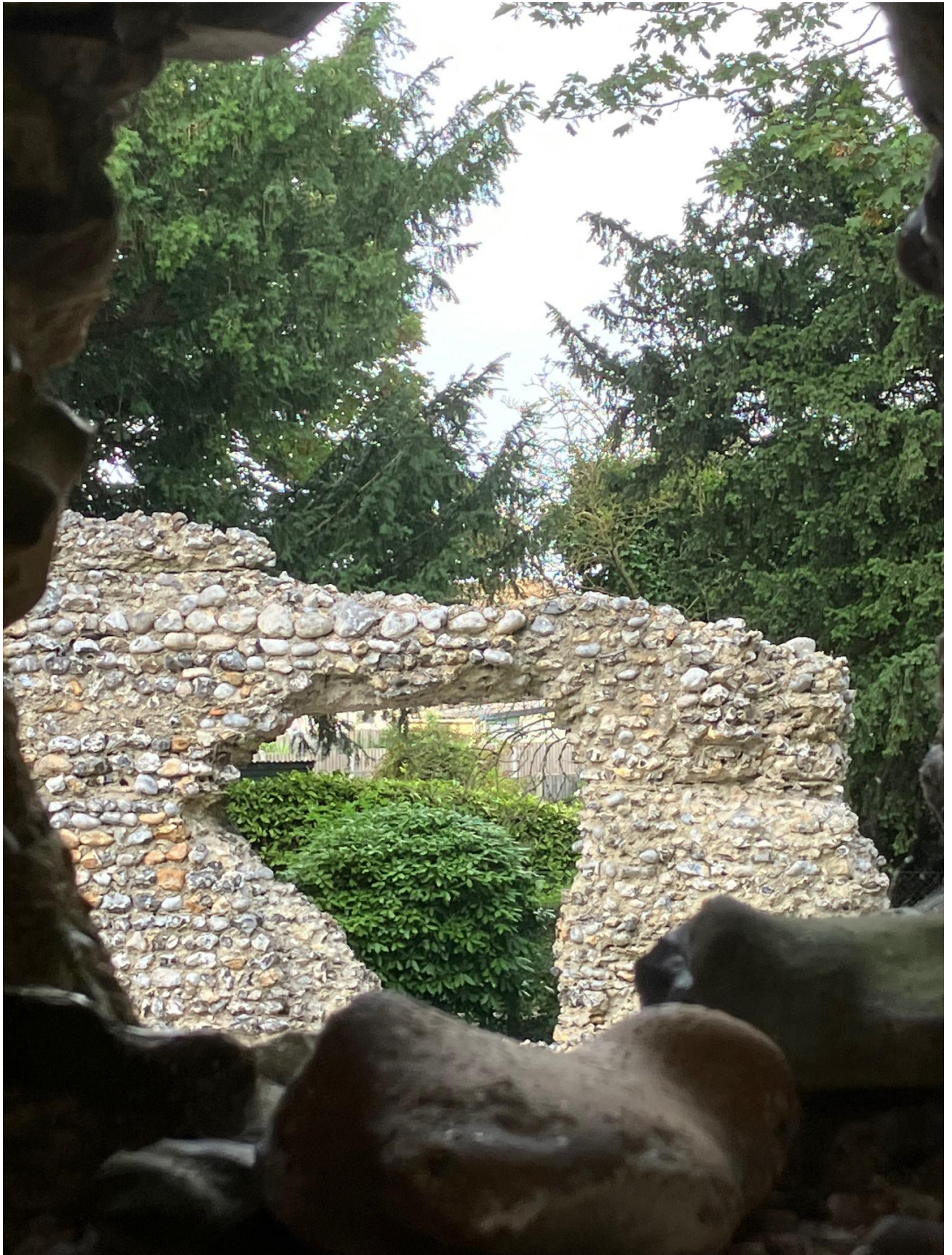
View of consolidated wall
