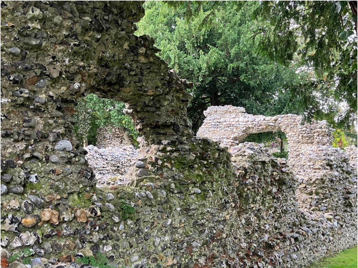
Various remaining walls within the keep area
