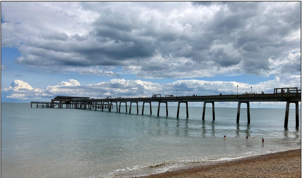
Fig. 55 The modern pier at Deal (built 1954, photo author, 2023).
