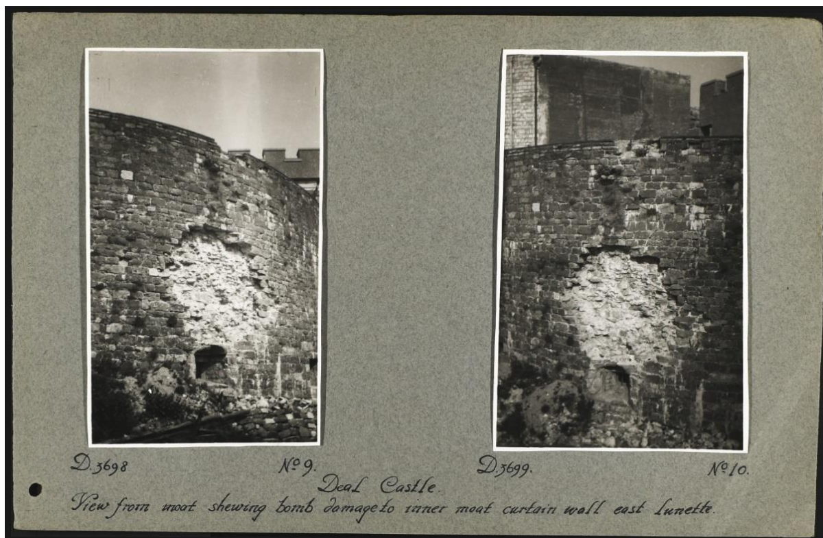
Fig. 43 Unpublished images of WW2 damage, April 1945, The National Archives, WORK/14/1943/118.
