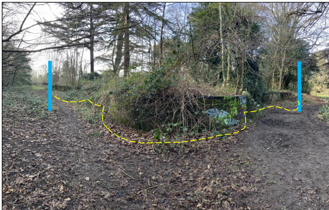
Fig. 31 Twentieth Century brickwork outlines the approximate location of the ruined Nonsuch Banqueting Hall, (photo author, 2024).
