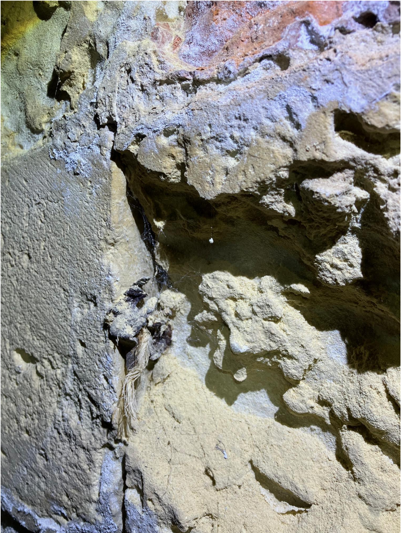
As with Camber Castle, The Rounds display many examples of honeycomb erosion. A former hammock hook and string is also present in the photograph.
