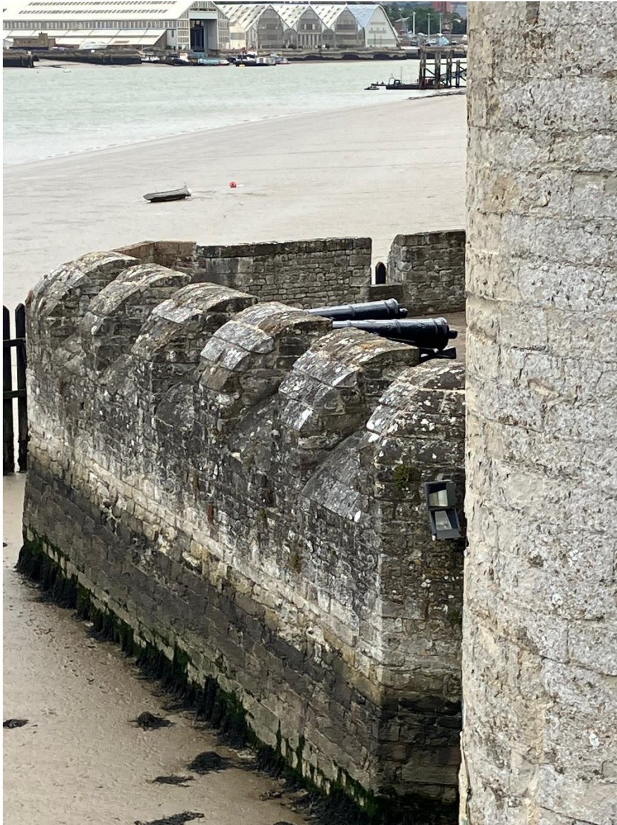
Rounded crenellations that defend against return fire are reminiscent of The Downs' embrasures (likely also as Kentish ragstone too)
