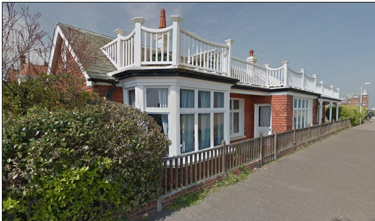
Fig. 15 Photograph by the author in 2021 of how Clanwilliam House looks today.
