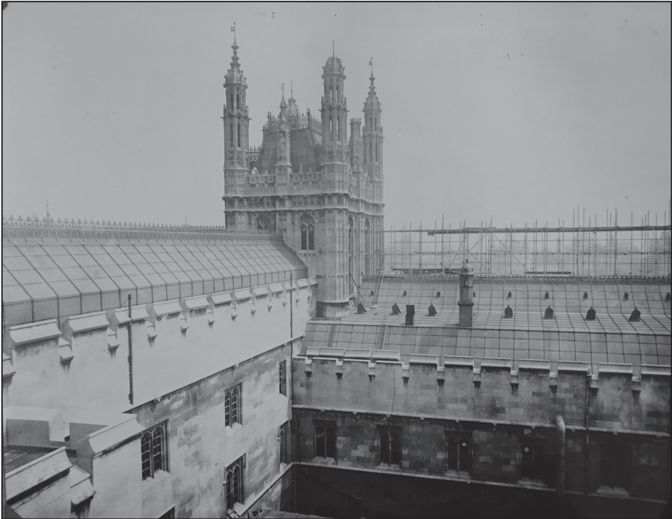
Figure 7: Photograph of original cast-iron roofs on the east and north side of Royal Court, taken c.1920s (Source: Historic England Archive, Swindon, AL 1016).
